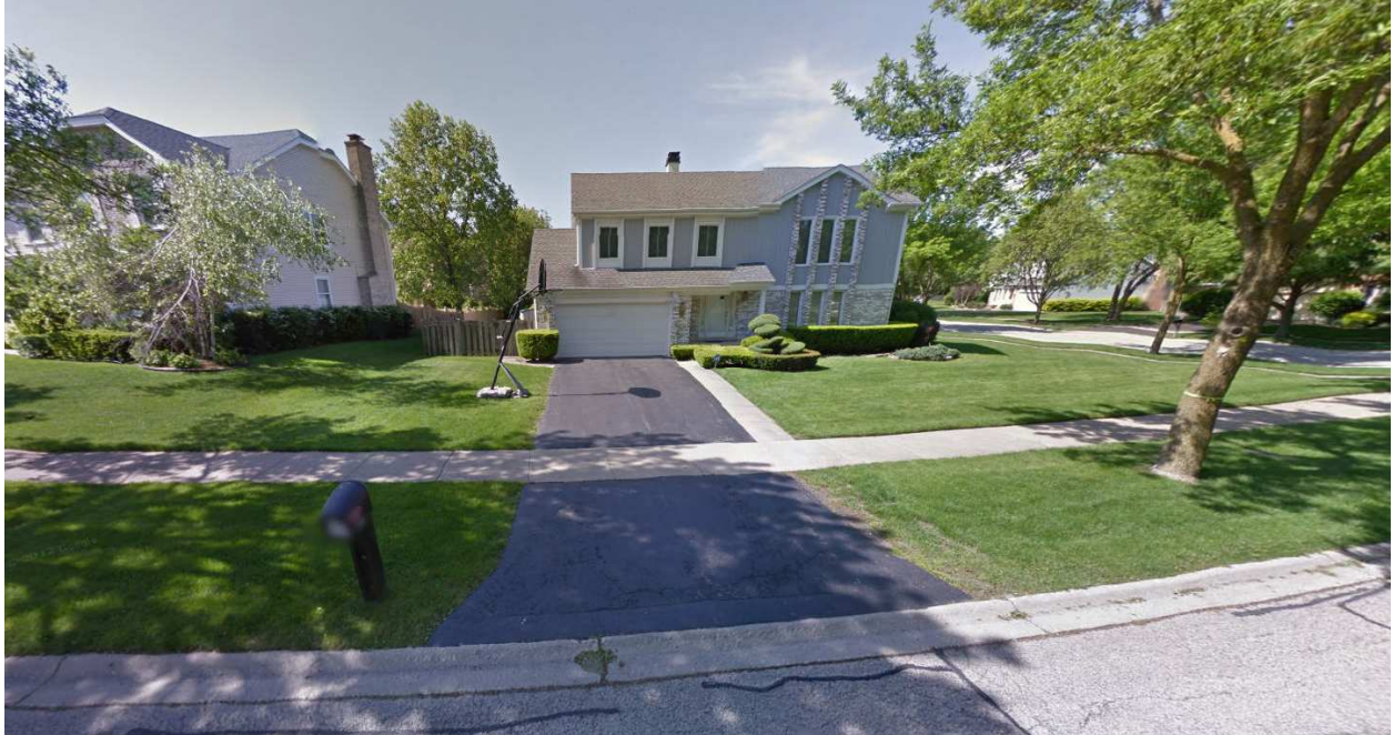
Photograph of Existing Structure
