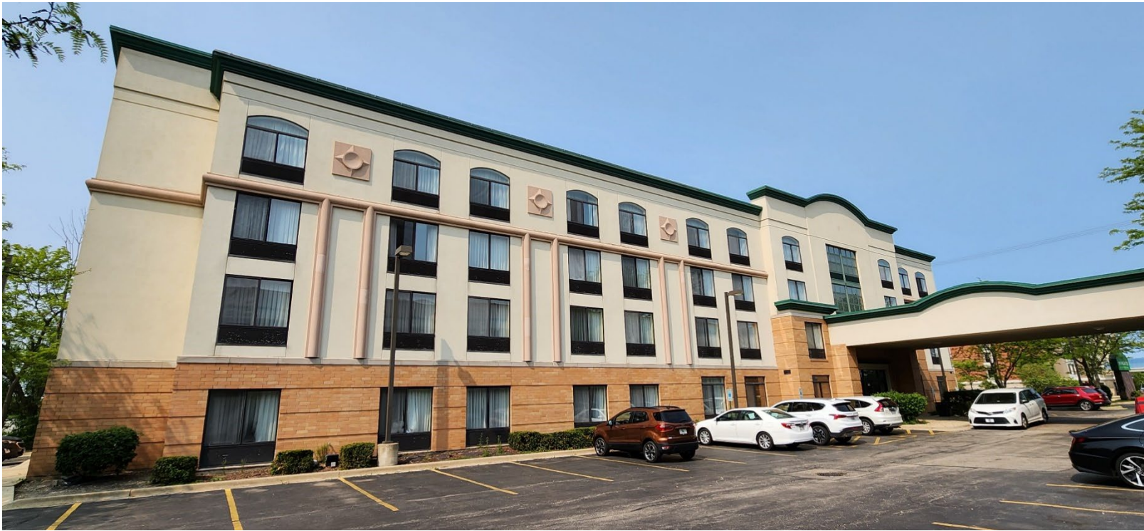
EXISTING SOUTH WALL
