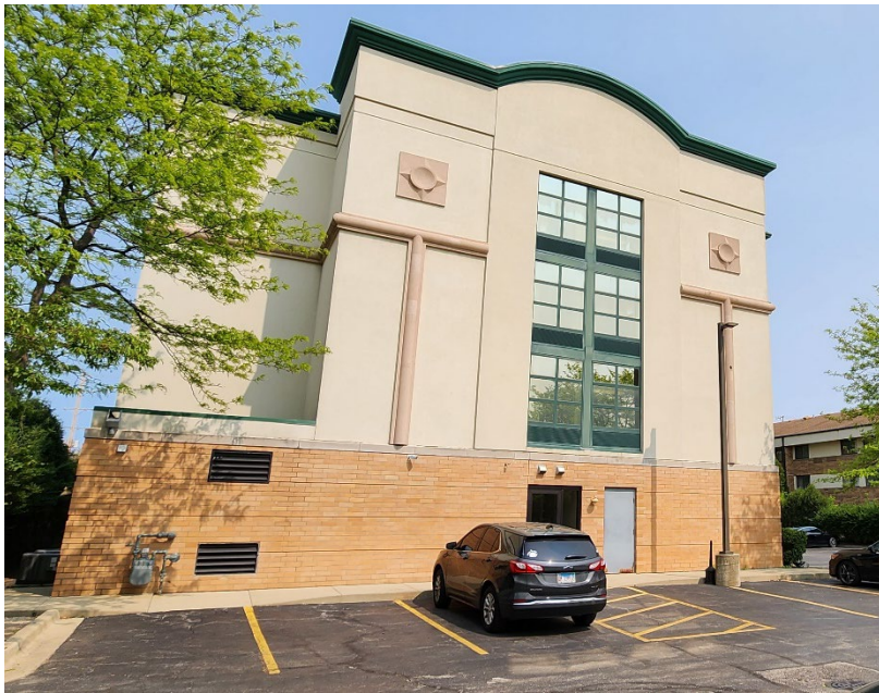
EXISTING WEST WALL
