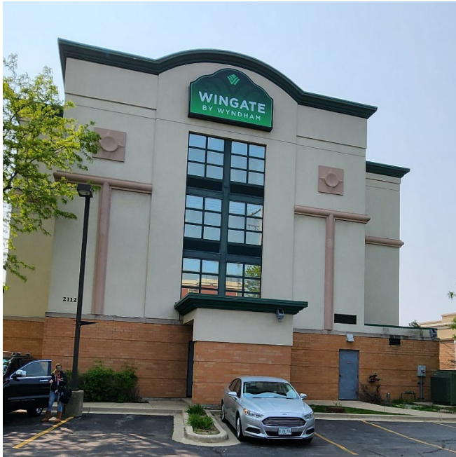
EXISTING EAST WALL
