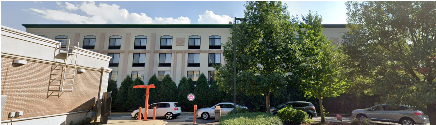
EXISTING NORTH WALL
