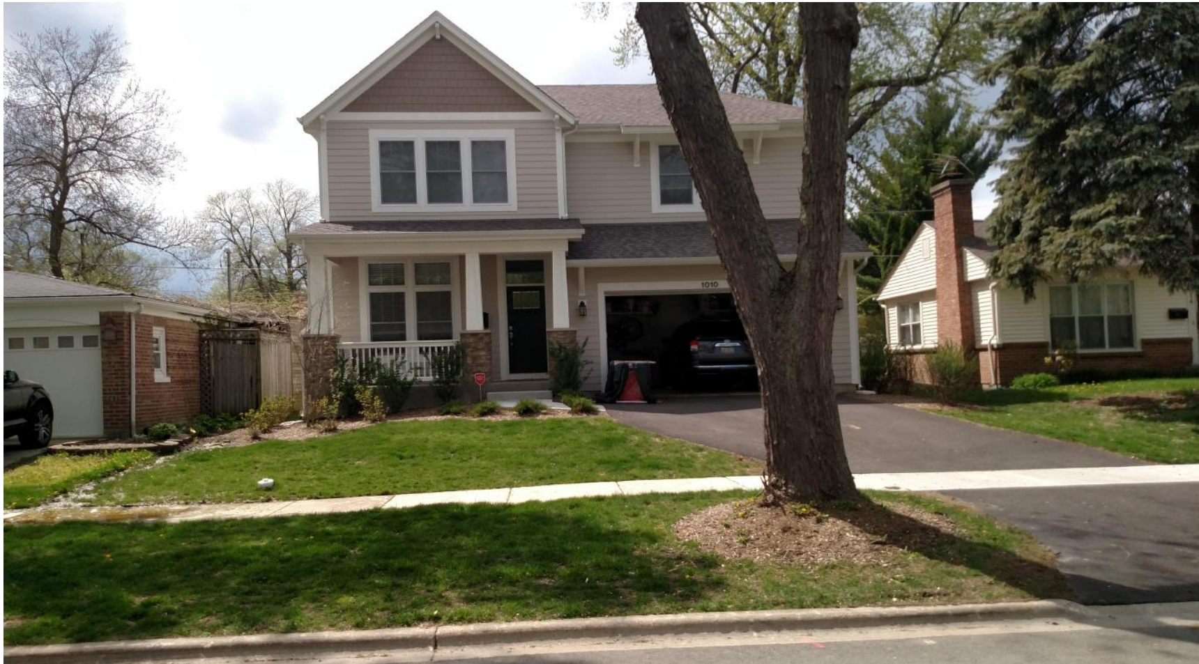
Existing House at 1010 N. Chicago Avenue
