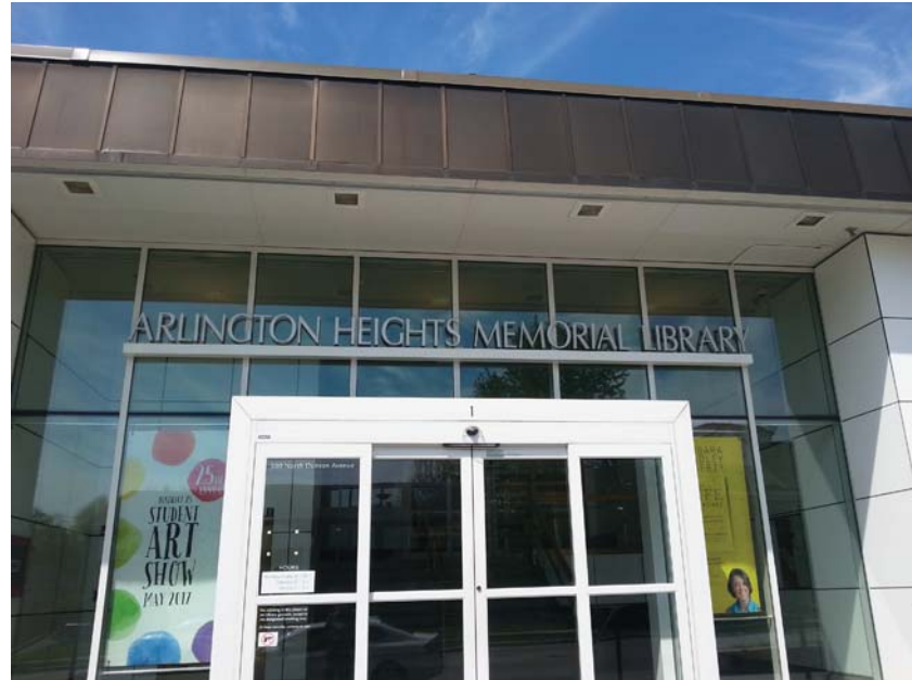
EXISTING EAST ELEVATION SIGNAGE (MAIN ENTRANCE)
