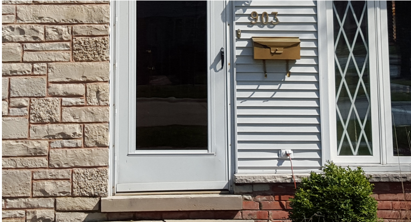
Close-up of existing stone, brick veneer, siding
