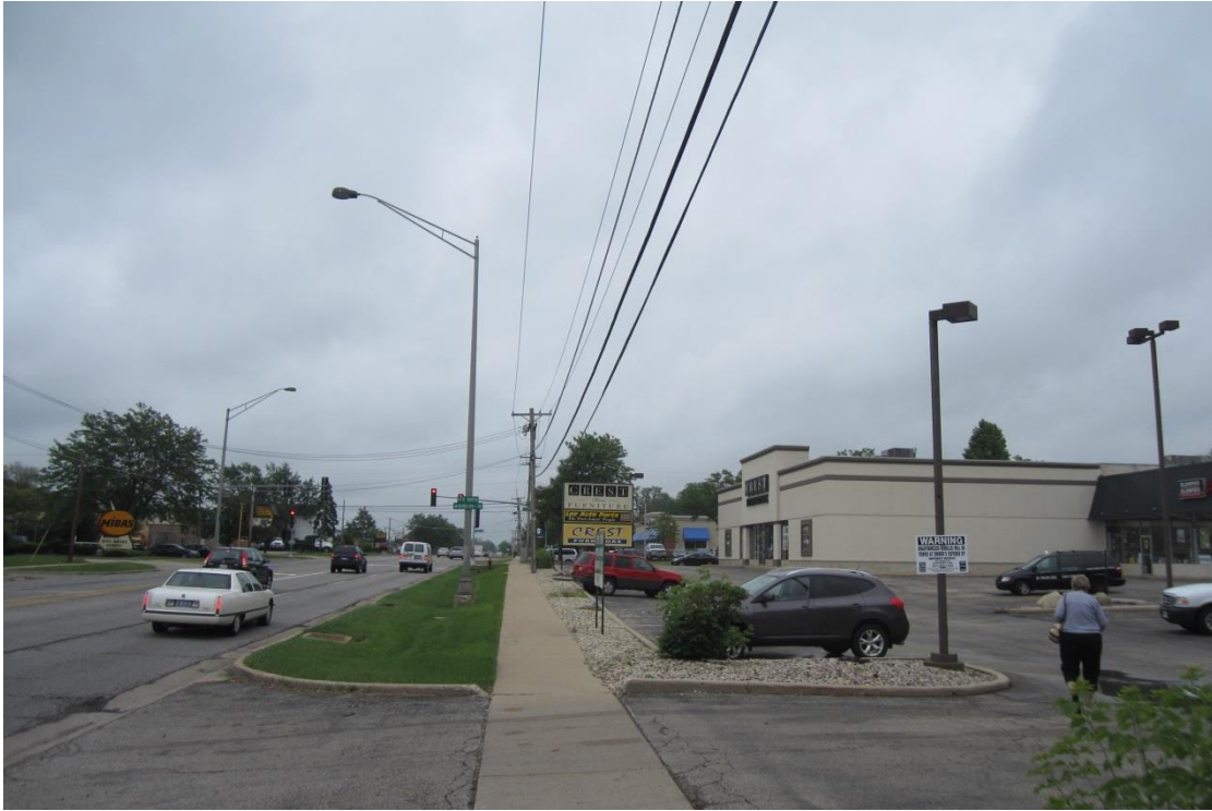
Photo 2 – view East from Northwest corner of property showing overhead power lines and sign in middle island along Rand Rd..
