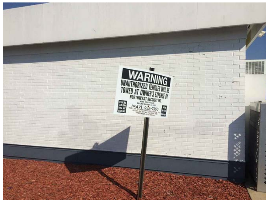
LEFT SIDE OF EXISTING BUILDING-View 2
