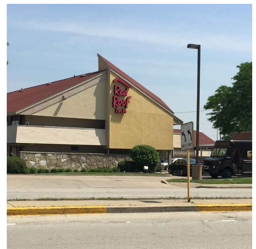
SURROUNDING PROPERTIES- View 10
