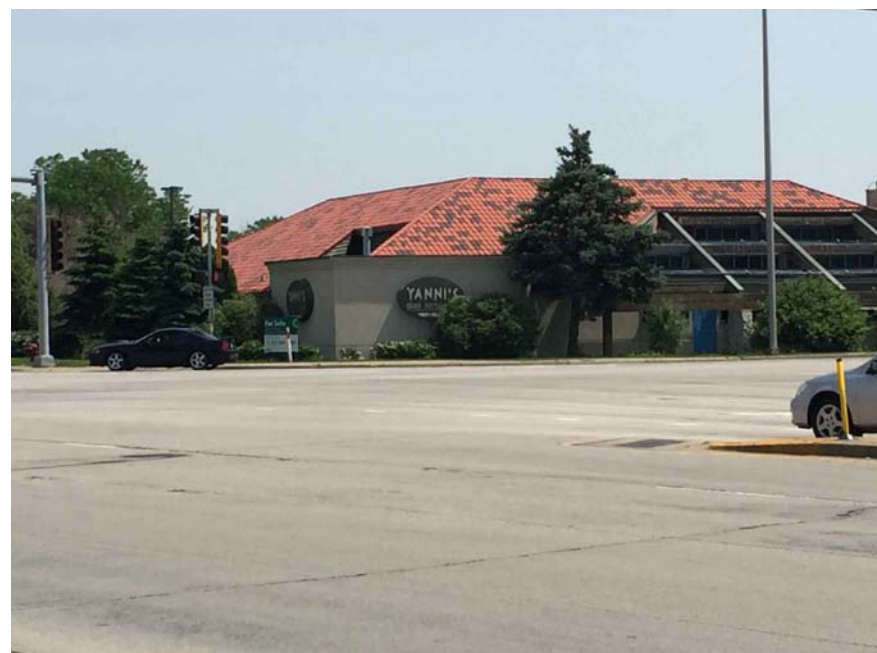
SURROUNDING PROPERTIES- View 9
