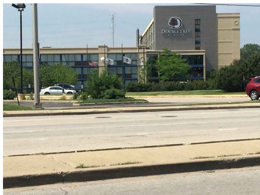
SURROUNDING PROPERTIES- View 5
