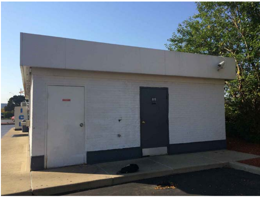
RIGHT SIDE OF EXISTING BUILDING - View 3
