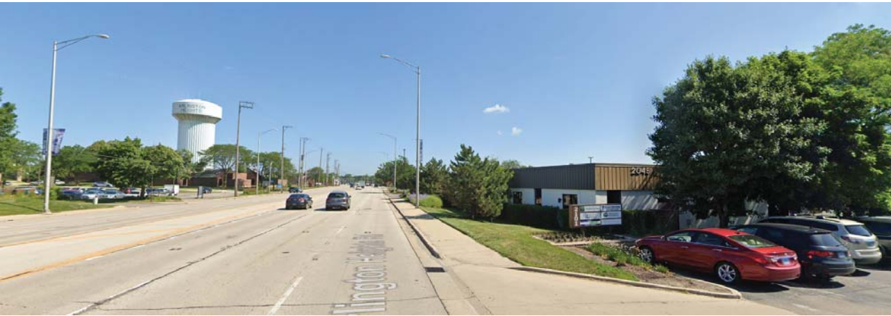
1 STREET VIEW - FROM SW CORNER, LOOKING NORTH
