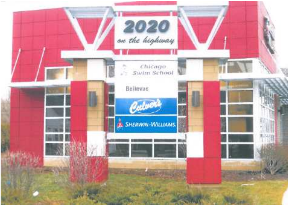
Photo of existing multi-tenant ground sign at west end of site.
