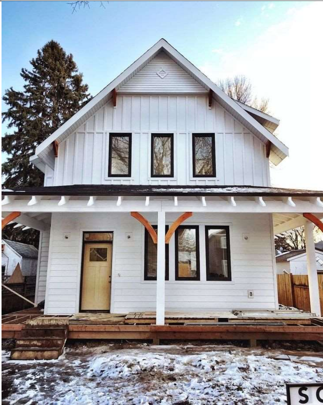
This is another example of vertical and horizontal siding being combined in the same elevation. Also note the color scheme is very close to what is proposed for 203 S Ridge.
