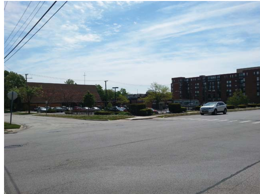
ADJACENT PROPERTY AT CORNER OF DUNTON AND ST. JAMES
