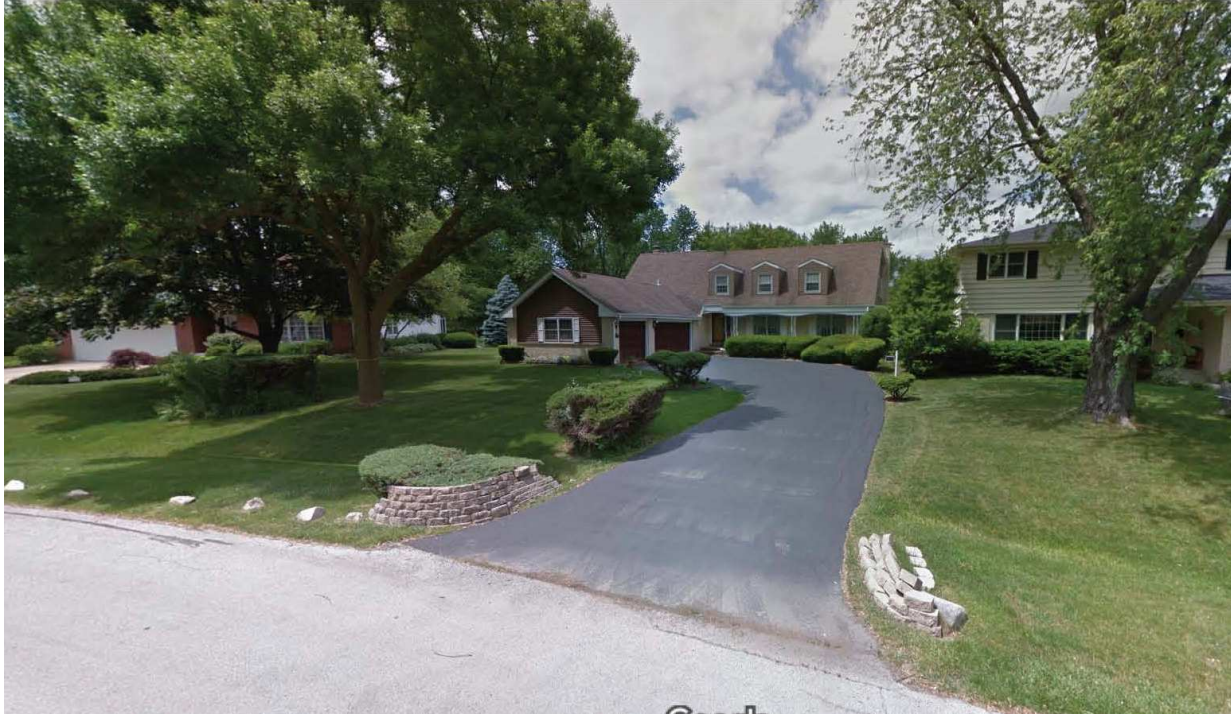
Photograph of Existing Structure
