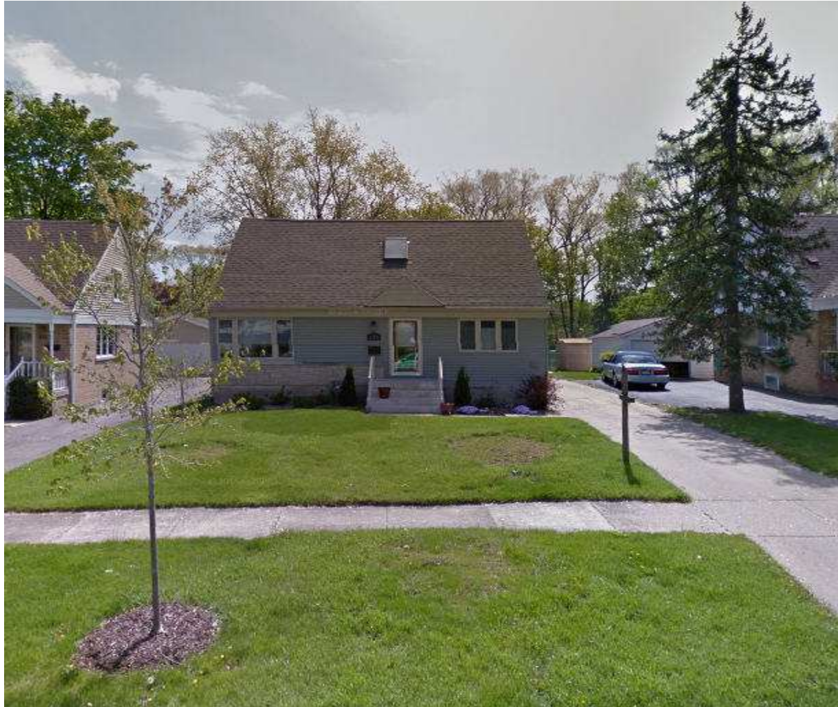
Photograph of Existing Structure
