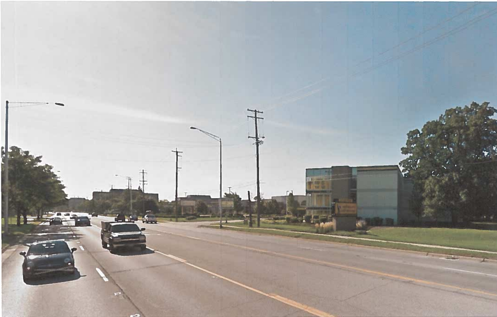
1st Building to West
