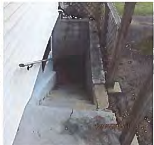
Repair path of egress/ingress. Replace guardrail and handrail at Basement staircase
