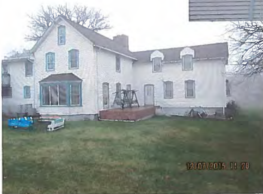
Low voltage and lightning rod wires draped throughout at exterior.
