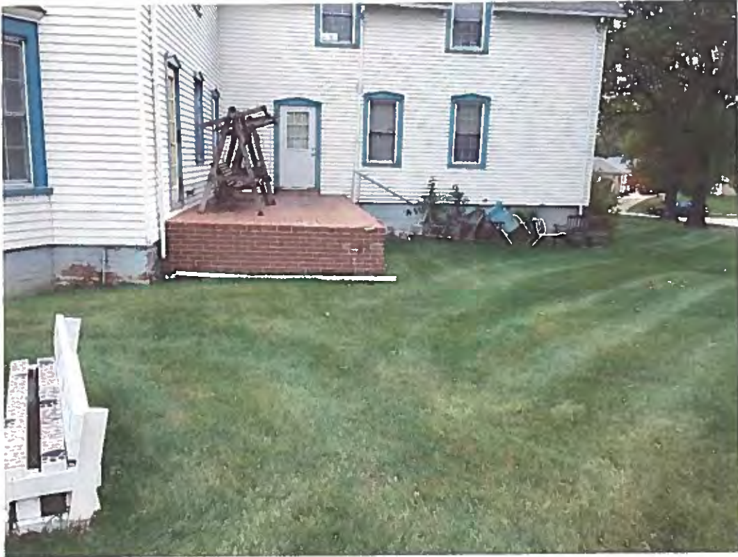
Install guardrail and replace stairs at rear patio. Tuck point basement brick walls.
