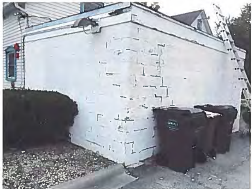
Animals entering main roof. Electrical conduit and lighting improperly installed. Siding damage. Separation of cinder block walls due to water damage. Damage at flat roof and fascia boards.
