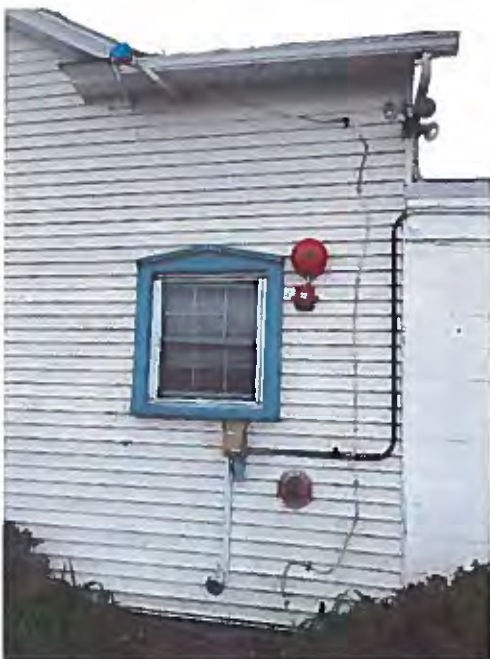
Animals entering main roof. Electrical conduit and lighting improperly installed. Siding damage. Separation of cinder block walls due to water damage. Damage at flat roof and fascia boards.
