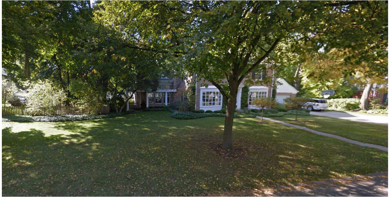
Photograph of Existing Structure
