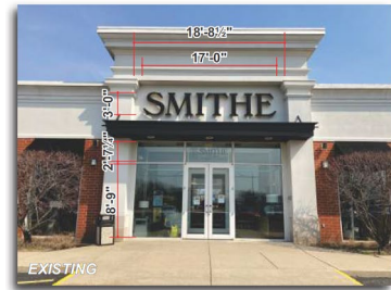
Southwest Elevation - Sign#6 - Before
