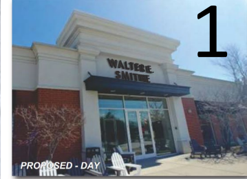
Southwest Elevation - Sign#1 - AFTER
