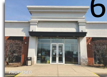
Southwest Elevation - Sign#6 - AFTER
