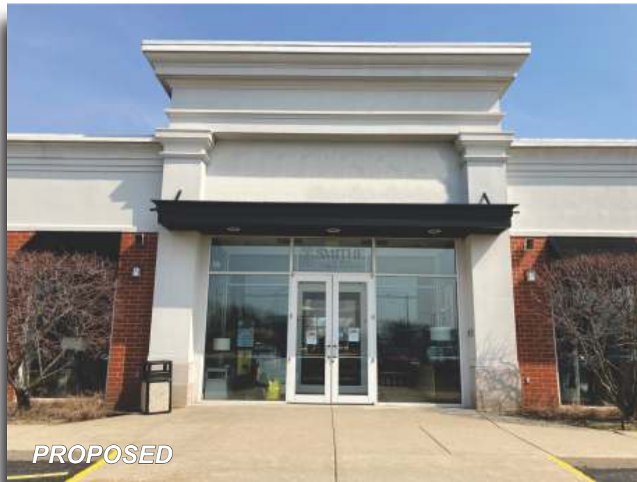
Southwest Elevation - Sign#6 - AFTER
