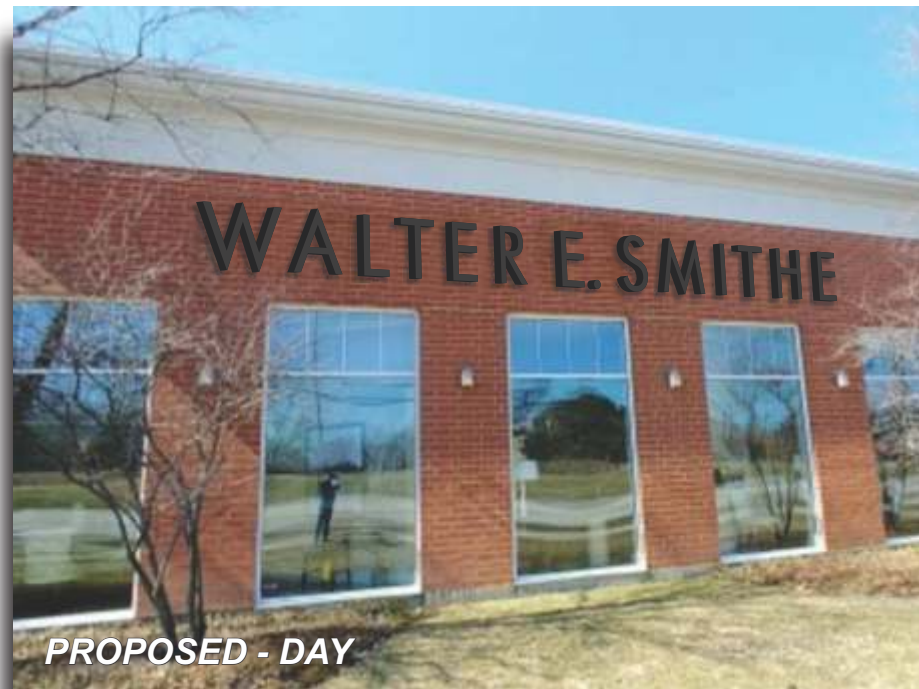
Northeast Elevation - Sign#3 - AFTER
