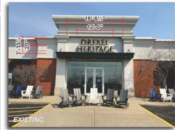
Southwest Elevation - Sign#1 - Before
