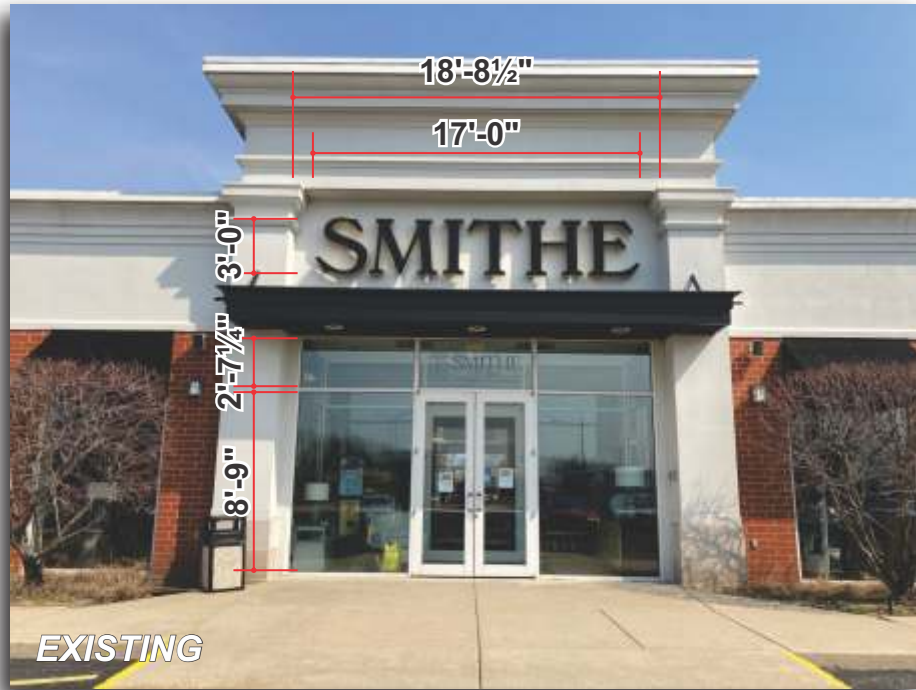
Southwest Elevation - Sign#6 - Before
