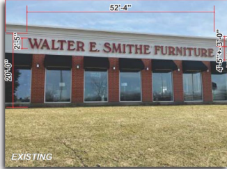
Northwest Elevation - Sign#4 - Before
