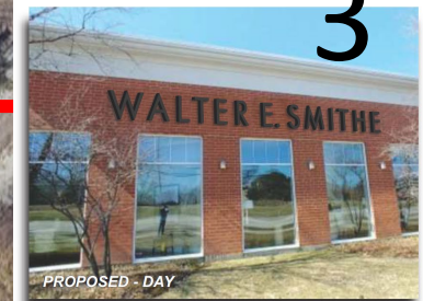
Northeast Elevation - Sign#3 - AFTER
