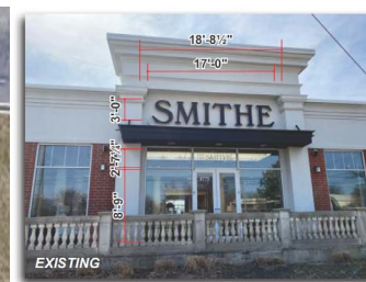
Northwest Elevation - Sign#5 - Before
