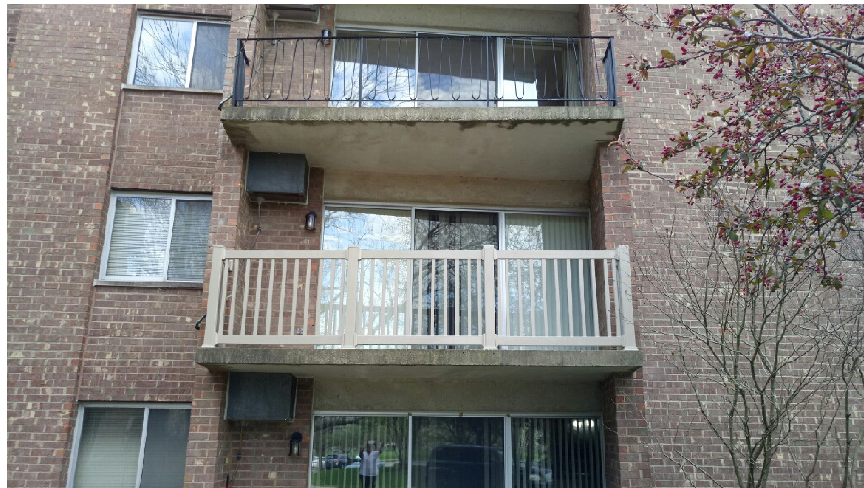
Stonebridge Apartment Buildings - Existing Site Photos / Railing Mockup
