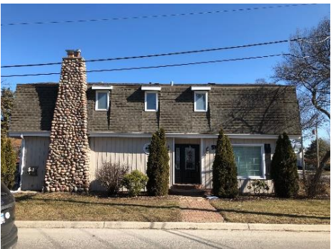
Property to left 1 5 N Ridge Ave
