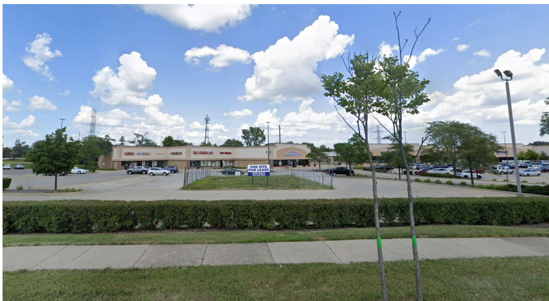
286 W Rand Road W Rand Road Looking Northeast
