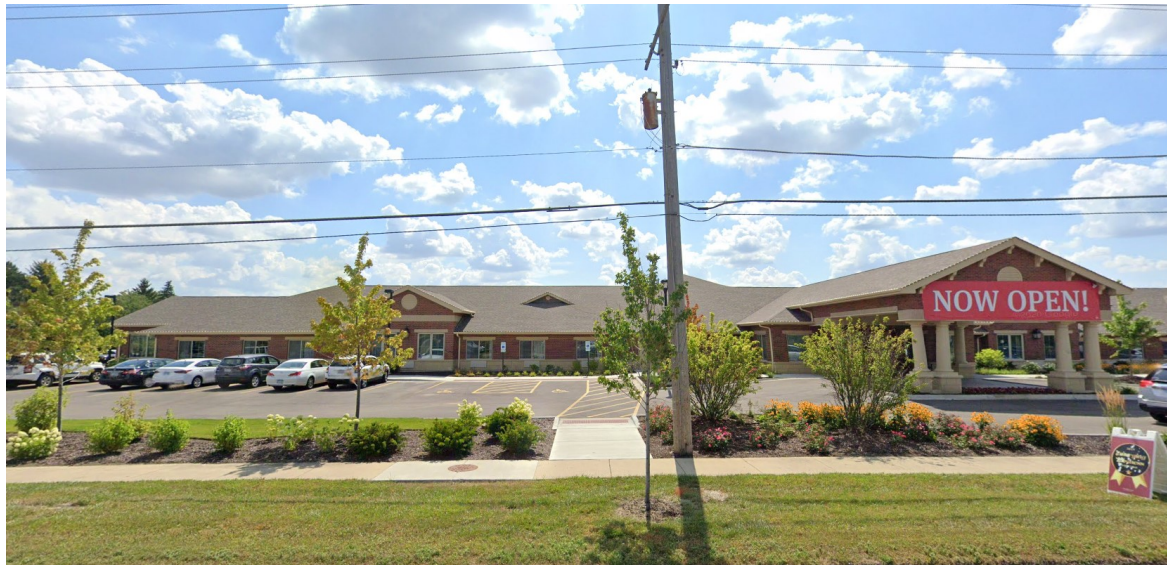
250 W Rand Road W Rand Road Looking Northeast
