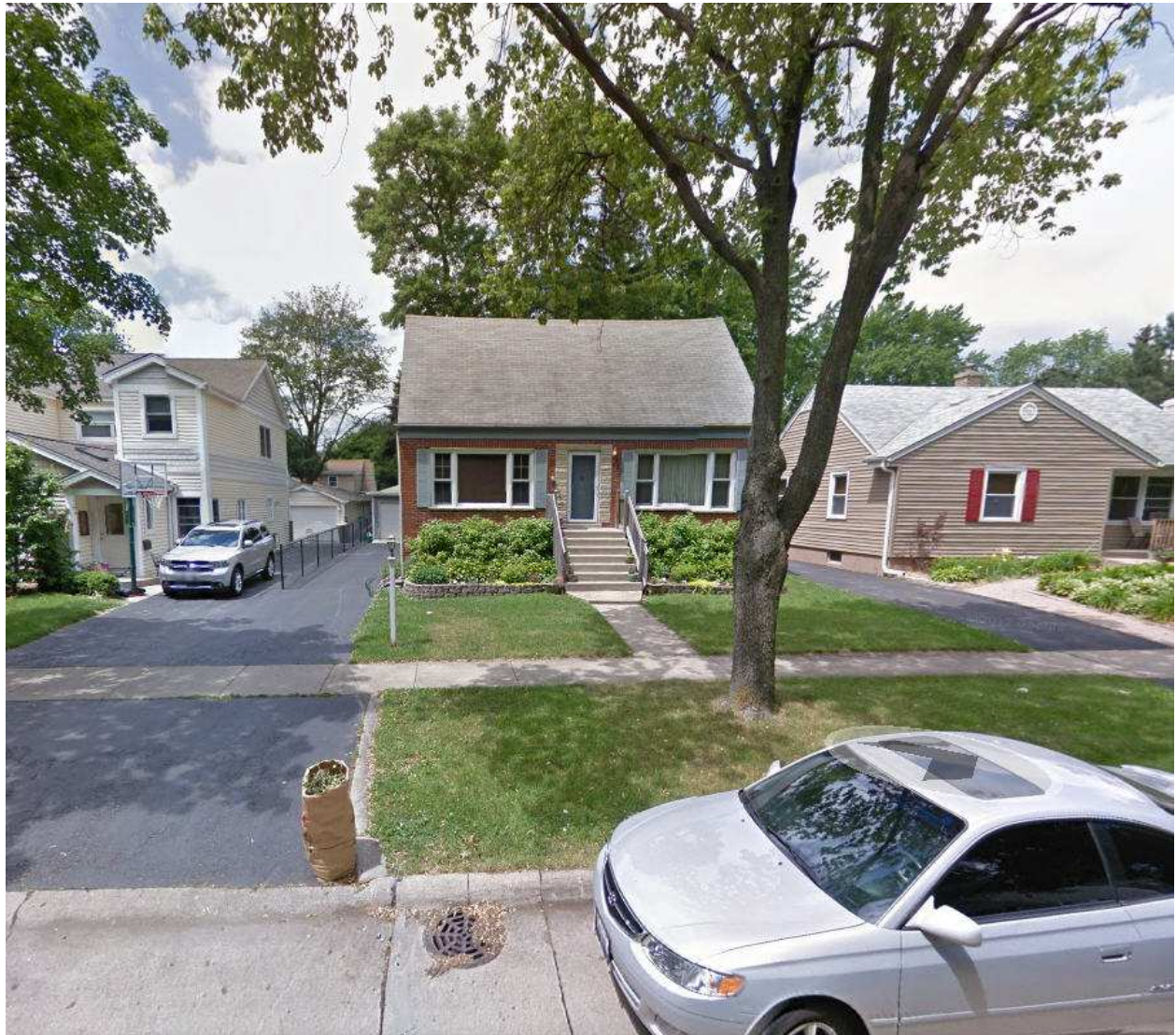
Photograph of Existing Structure
