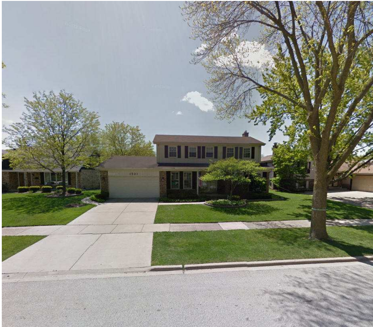
Photograph of Existing Structure
