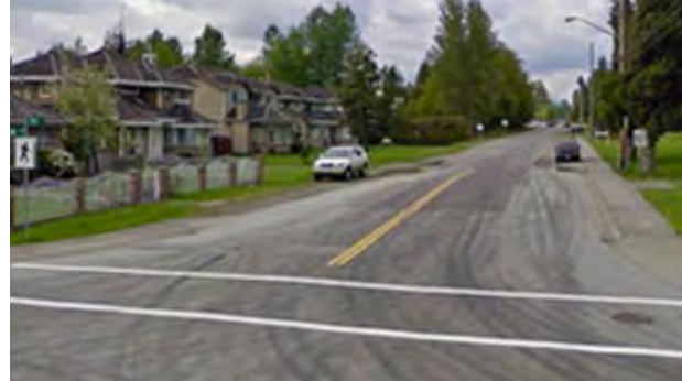
Figure 4.81 - Example A: Parallel Lines Crosswalk
