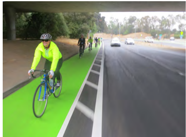
Figure 4.42 - Buffered Bike Lane (Green)
