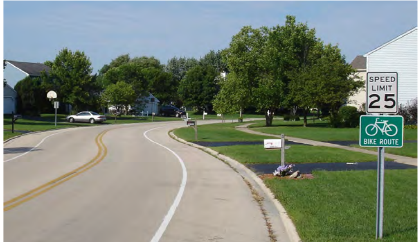
Figure 4.66 - Combined bicycle-parking lane in Warrenville, IL
