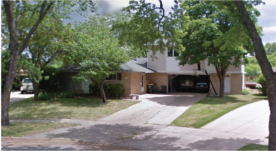
Photograph of Existing Structure
