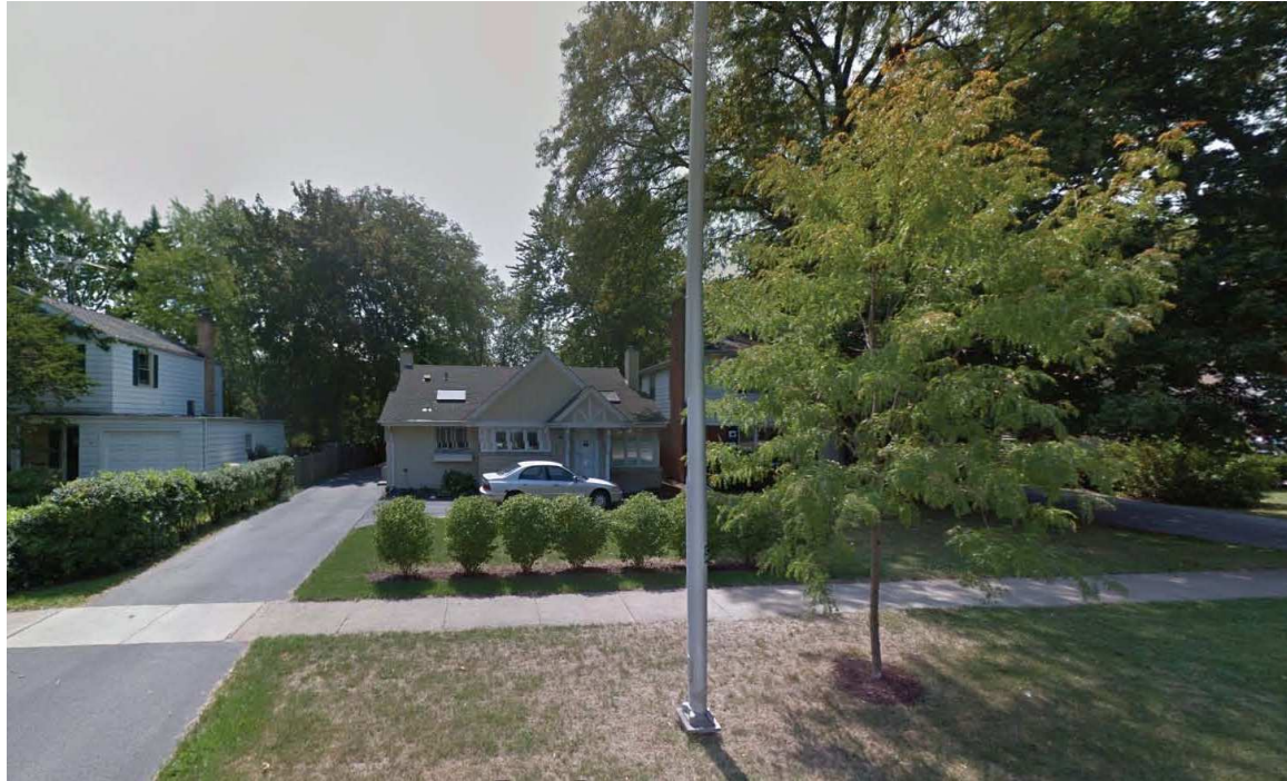
Photograph of Existing Structure
