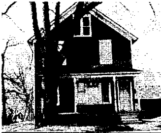
204 S. Arlington Heights Rd. DEMOLISHED
