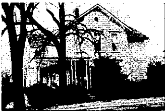
210 S. Arlington Heights Rd. DEMOLISHED
