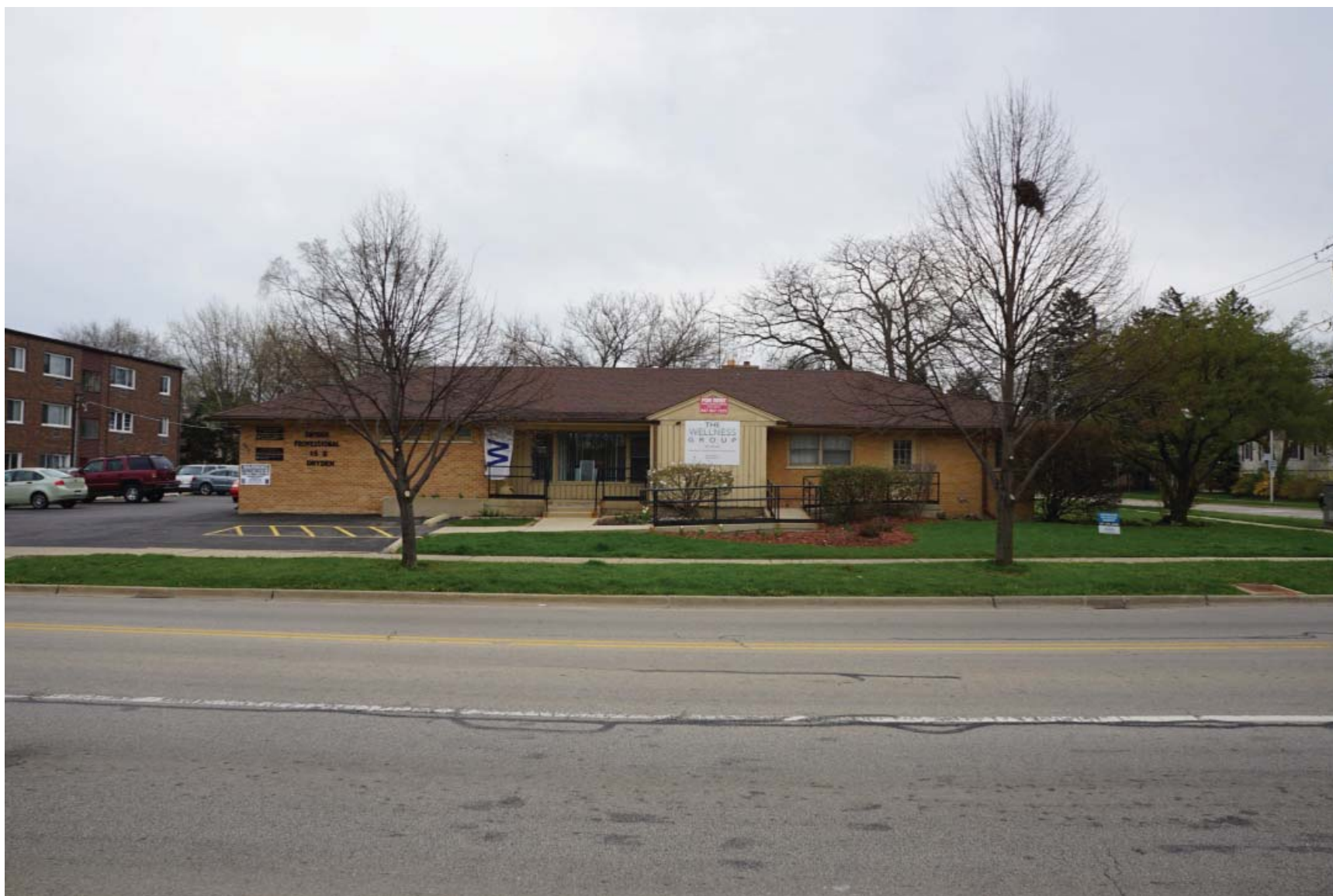
VIEW EAST OF KENSINGTON SCHOOL ON DRYDEN
