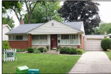
PROPERTY TO SOUTH 2 411 N HICKORY AVE
