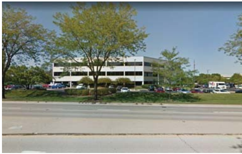
FIRST PROPERTY TO THE EAST
