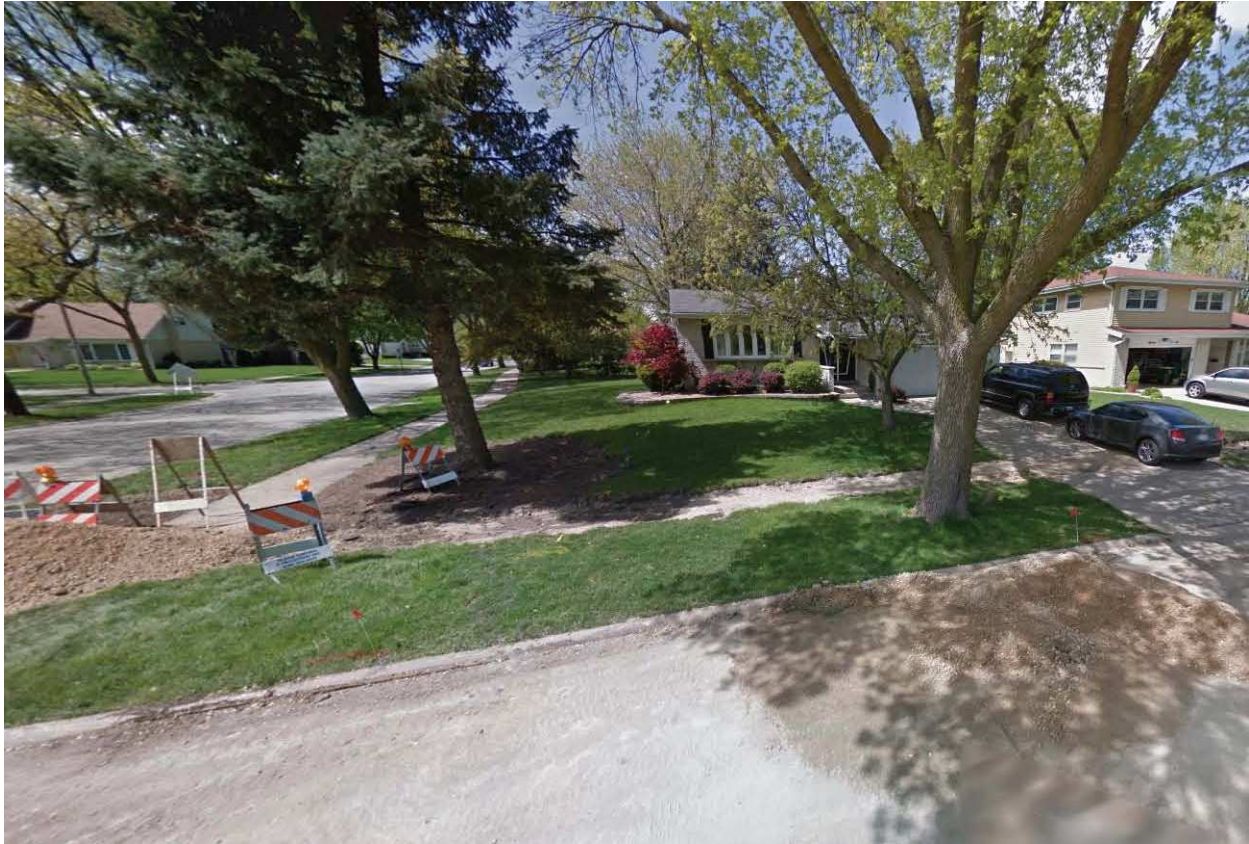
Photograph of Existing Structure
