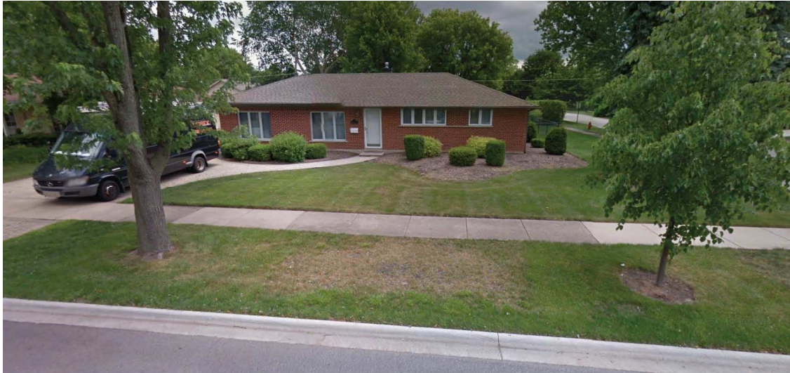
Photograph of Existing Structure
