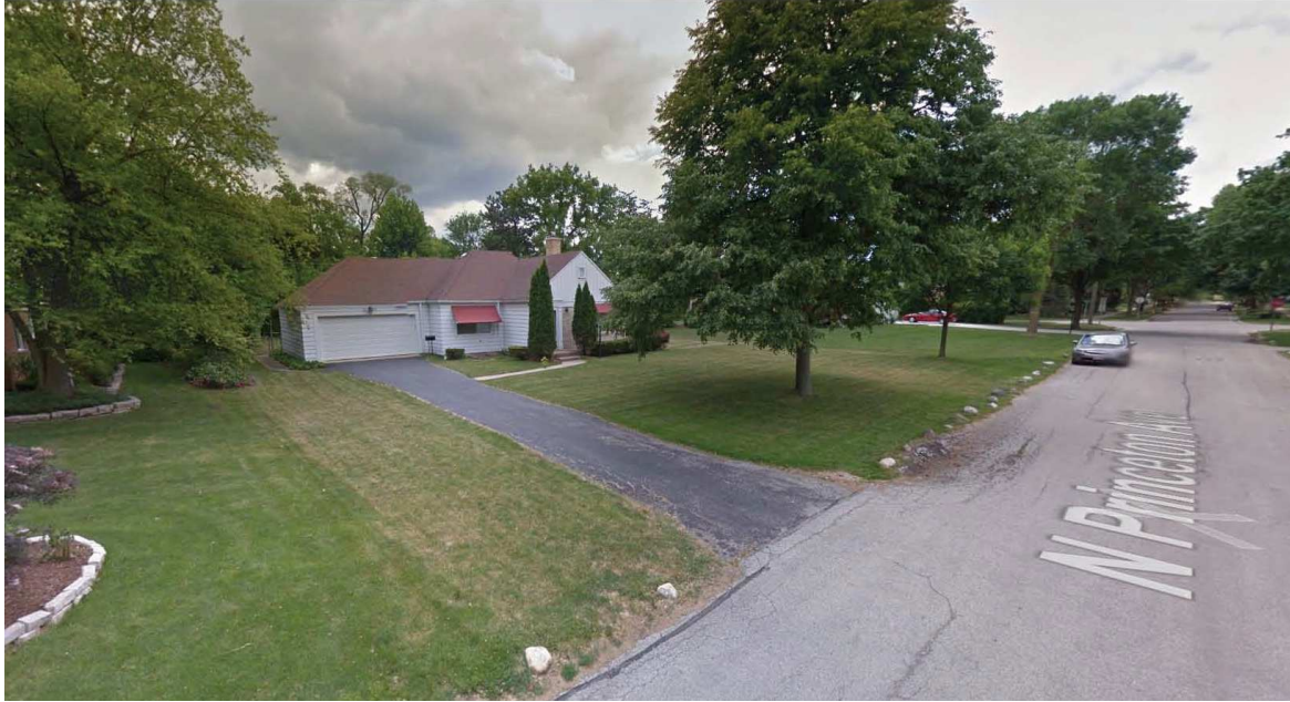
Photograph of Existing Structure
