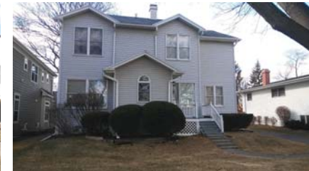
Property Across 5 922 S. Dunton Ave.
