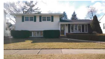
Property Across 4 920 S. Dunton Ave.
