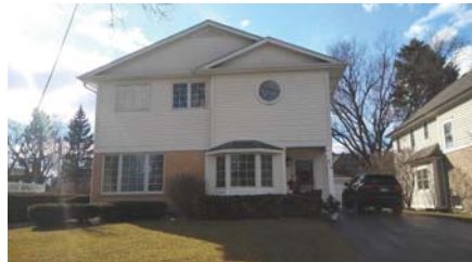
Property Across 2 914 S. Dunton Ave.
