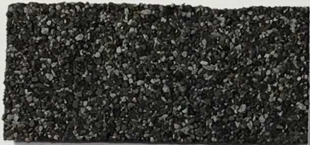
MAIN ROOF SHINGLE
