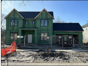
PROPERTY TO RIGHT #1 1200 N RACE AVE (UNDERCONSTRUCTION)
