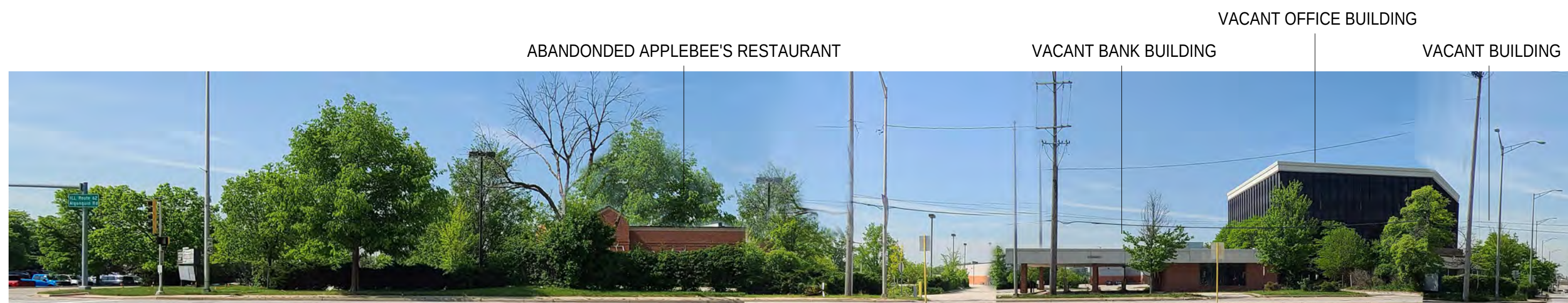
VIEW 8 - SOUTH VIEW - EAST ALGONQUIN RD
