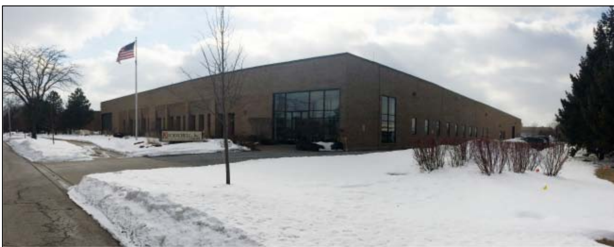
7 Building Photo Scale: NTS
