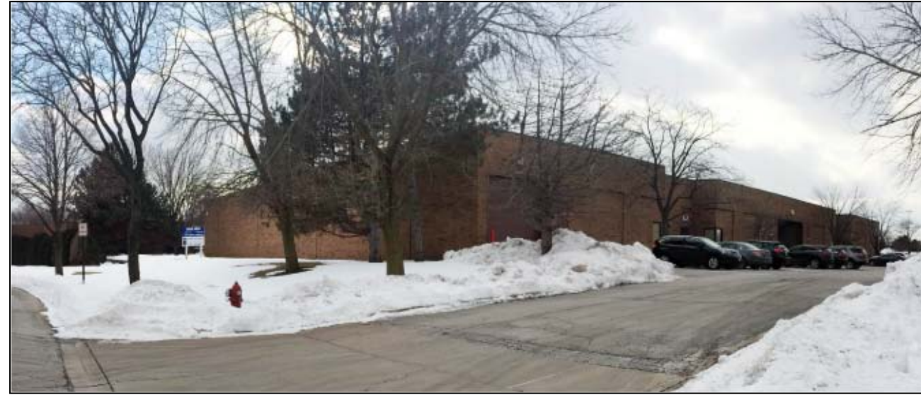
9 Building Photo Scale: NTS
