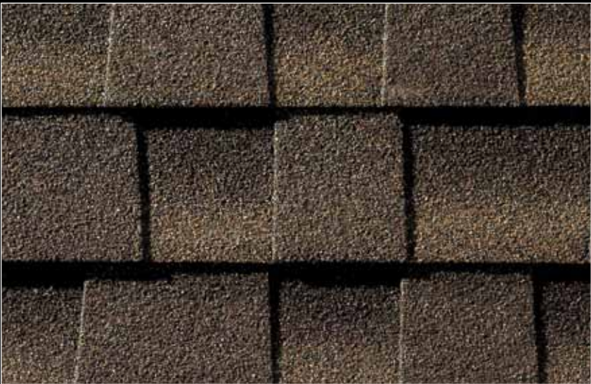
30-YEAR ROOF Barkwood
