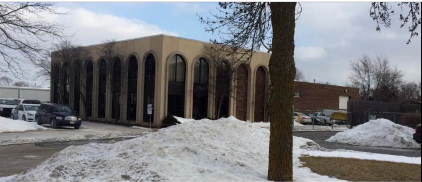
12 Building Photo Scale: NTS
