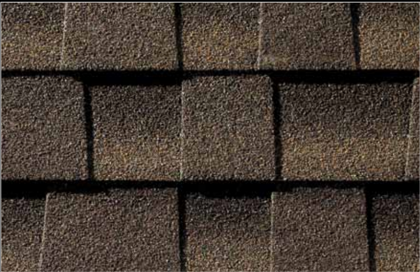
30-YEAR ROOF Barkwood
