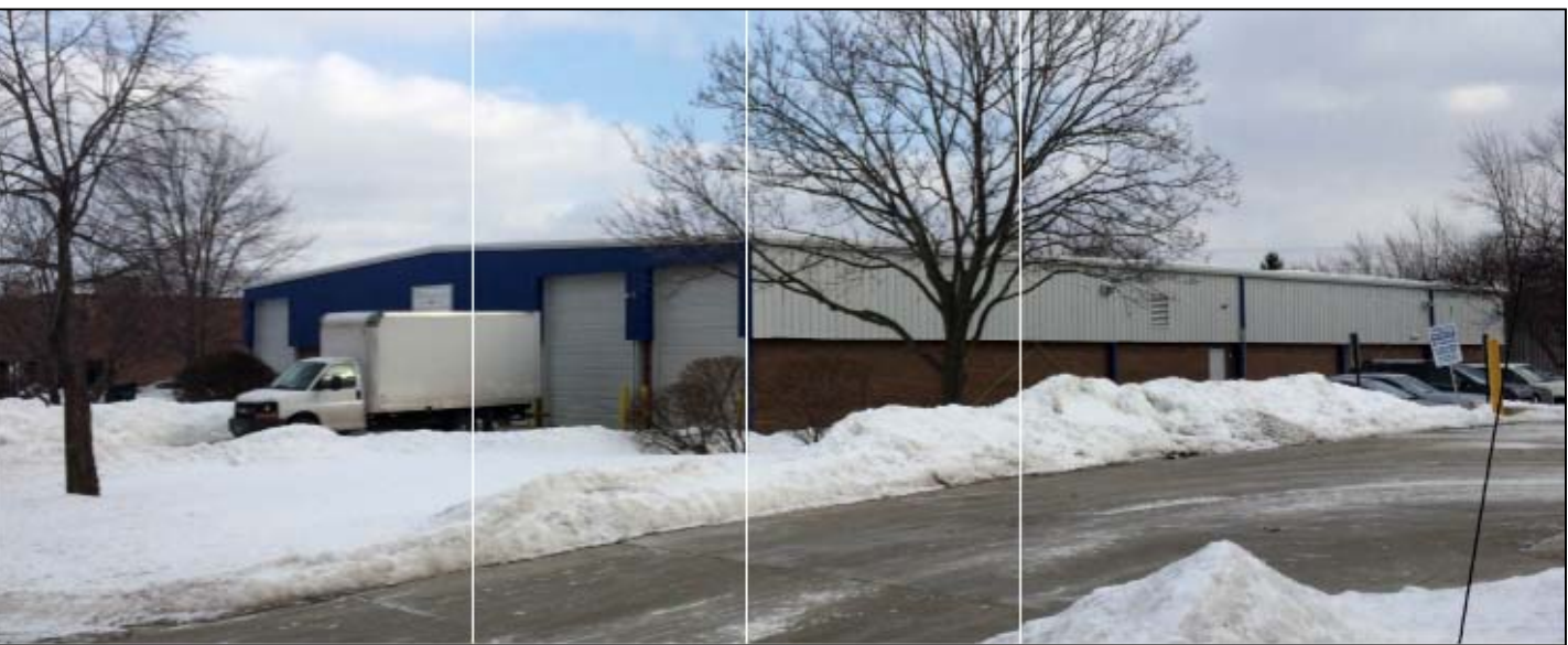
13 Building Photo Scale: NTS
