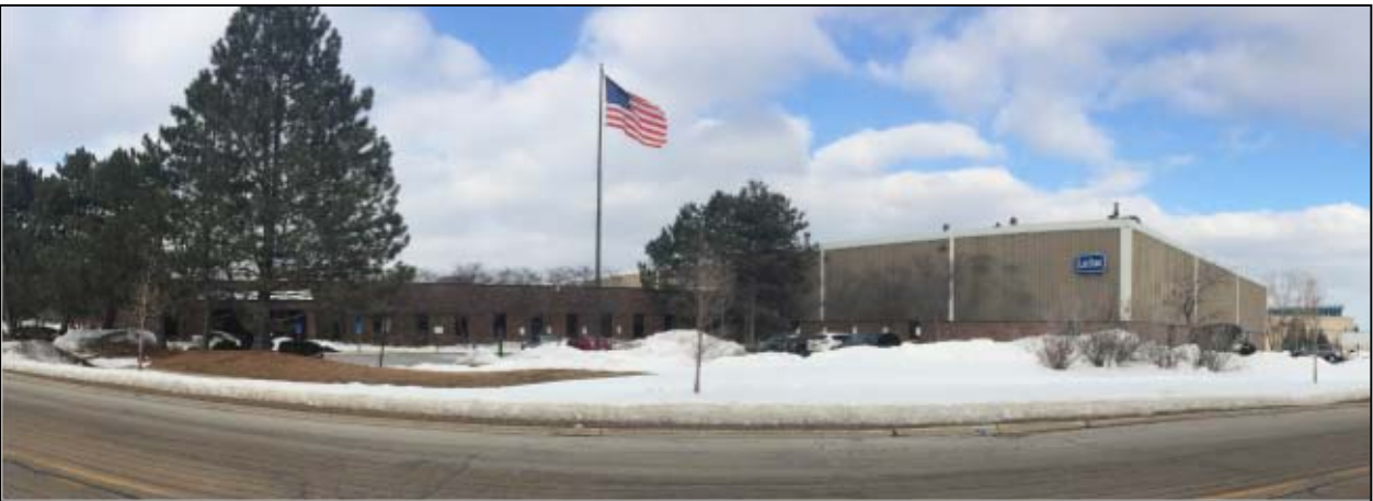
6 Building Photo Scale: NTS
