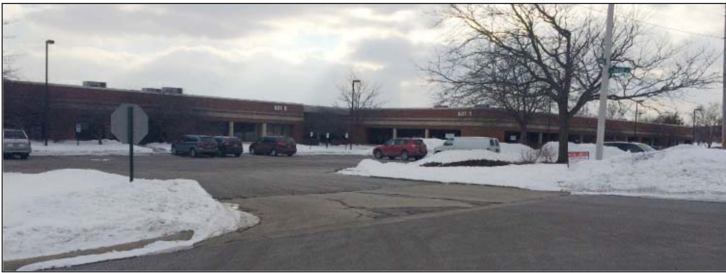
16 Building Photo Scale: NTS
