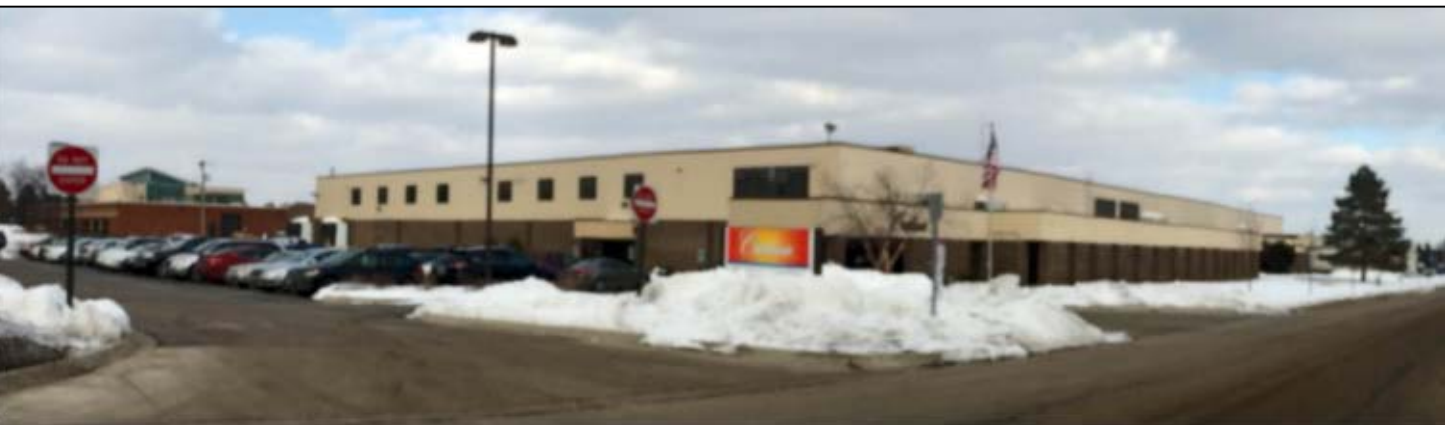
14 Building Photo Scale: NTS
