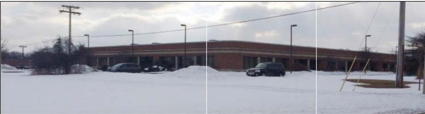
15 Building Photo Scale: NTS
