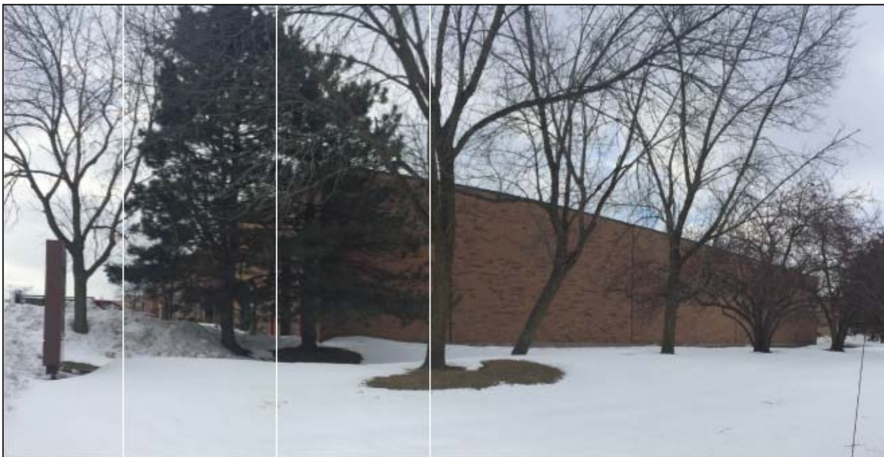
8 Building Photo Scale: NTS
