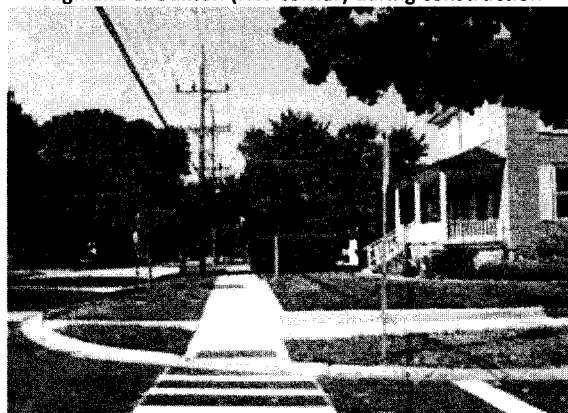
Highland & Oakton (NW corner) after retaining wall
