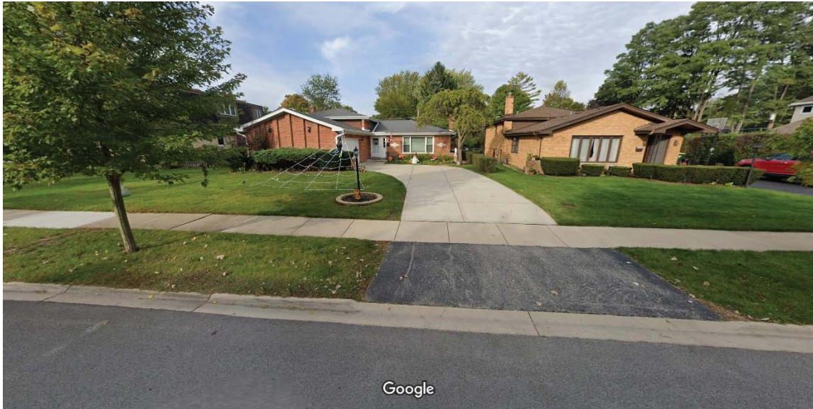
Photograph of Existing Structure
