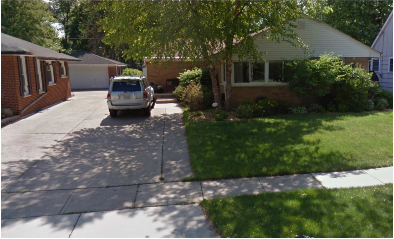
Photograph of Existing Structure
