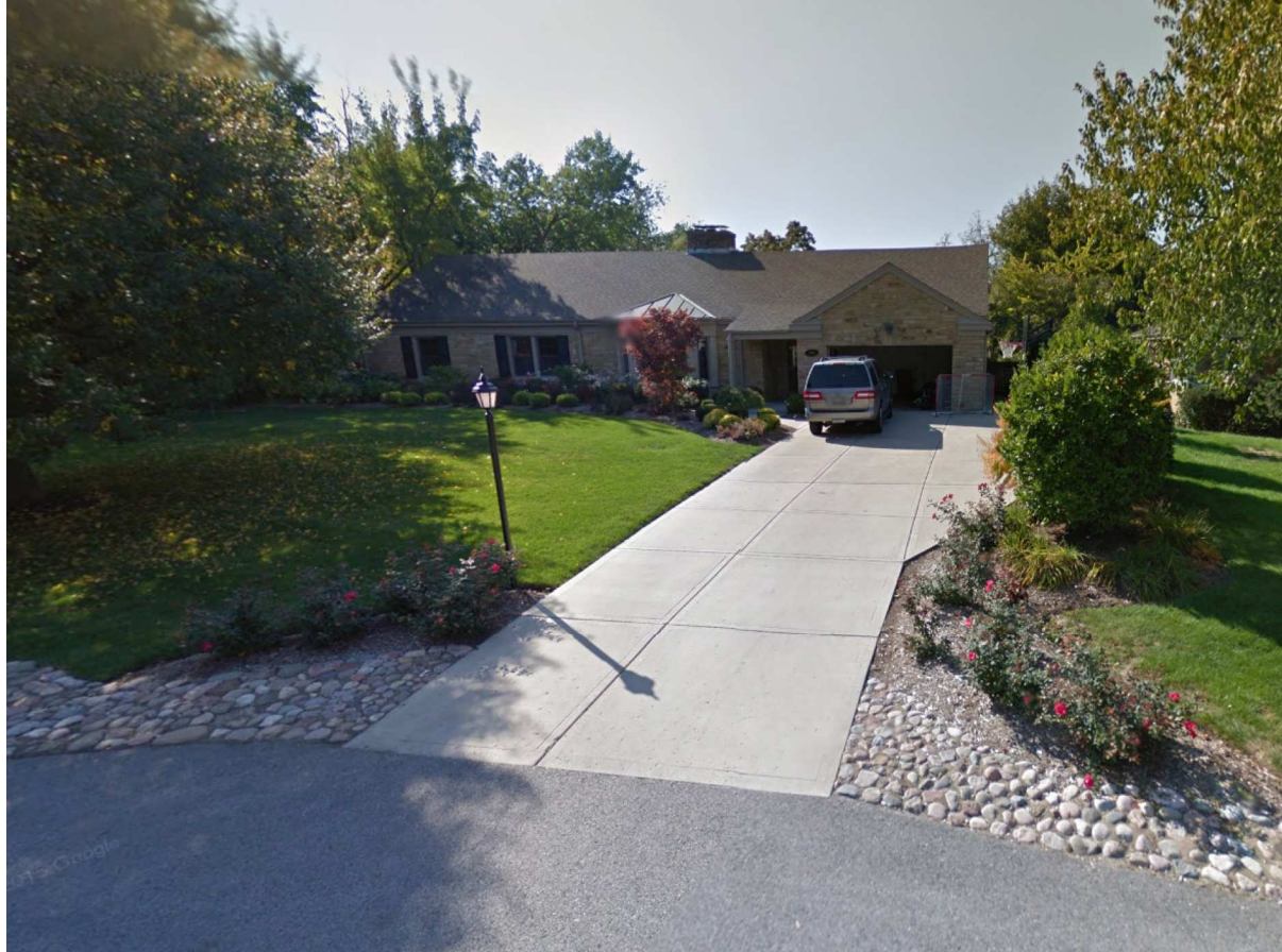
Photograph of Existing Structure
