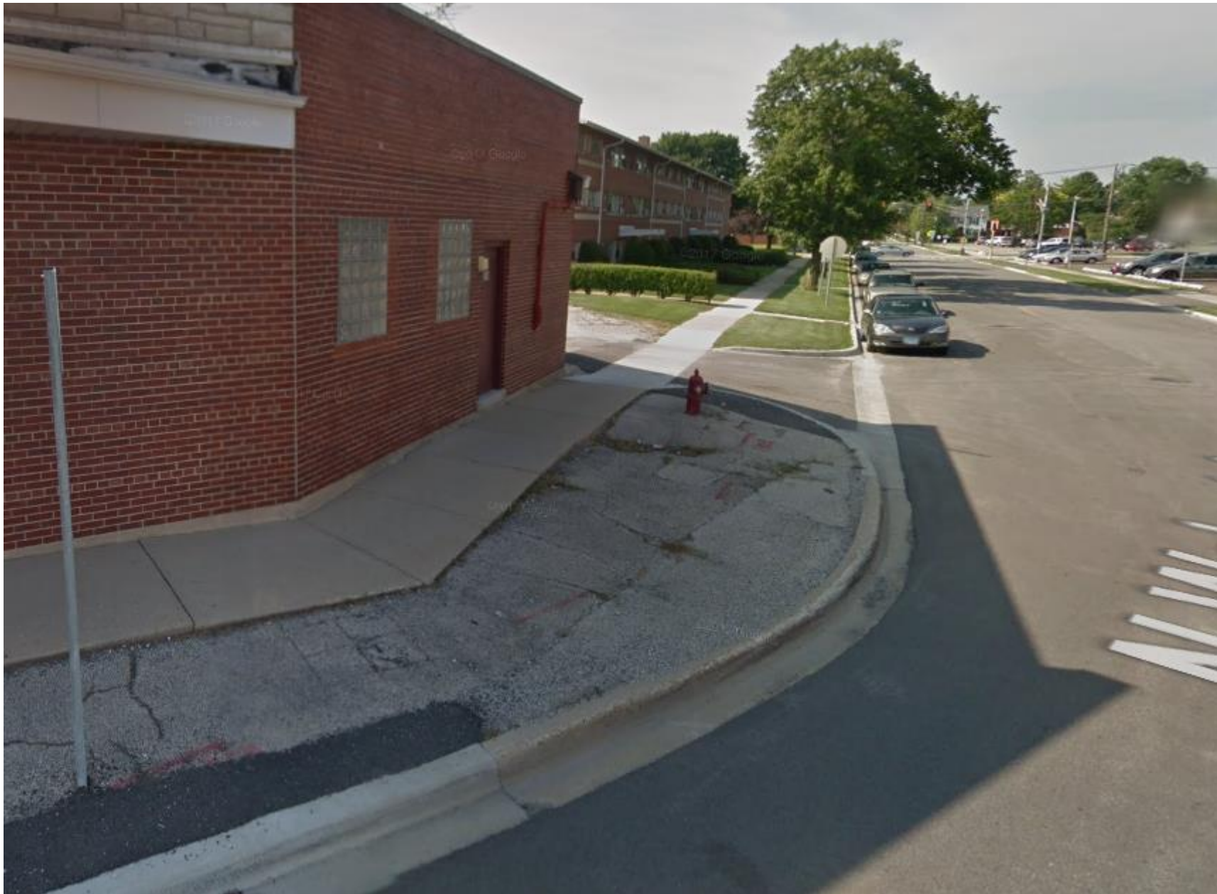
Asphalt Parkway at Walnut Avenue Looking North
