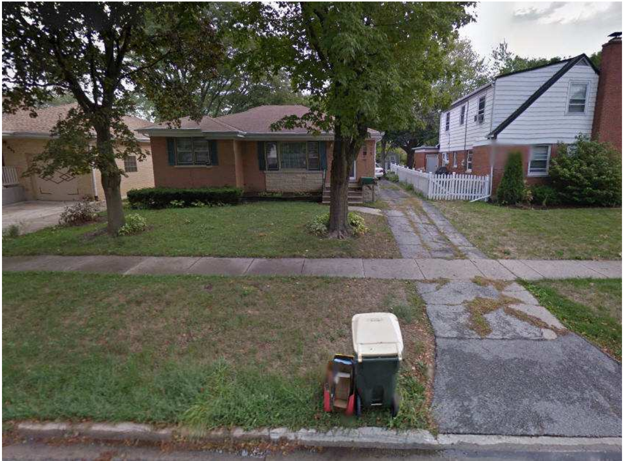
Photograph of Existing Structure
