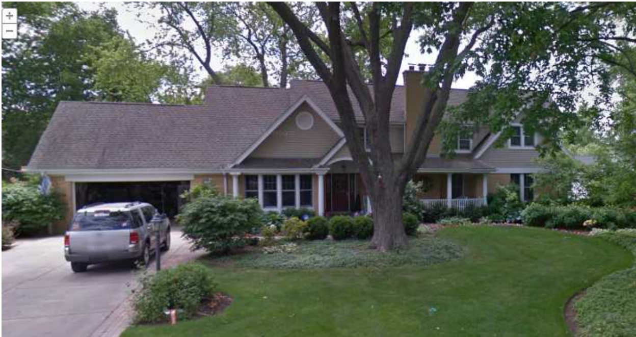
Image 1, 1303 W. Watling Street. This home is a very nice example of a second story addition to an existing single story house. The gable roof forms and front porch keep the scale of the expanded home within the context of the neighborhood.
