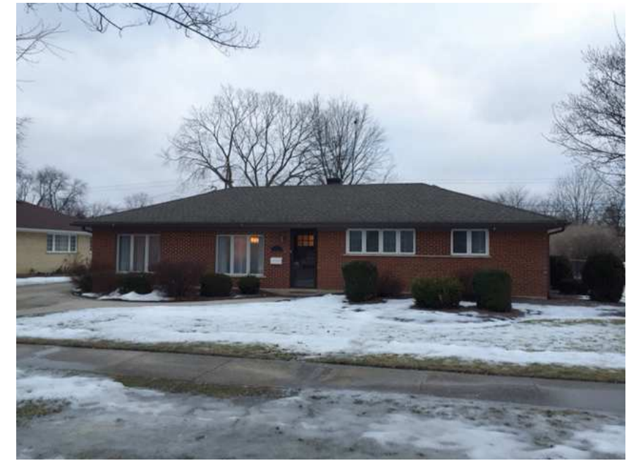
1605 N. Chestnut – Existing West Elevation Subject Property
