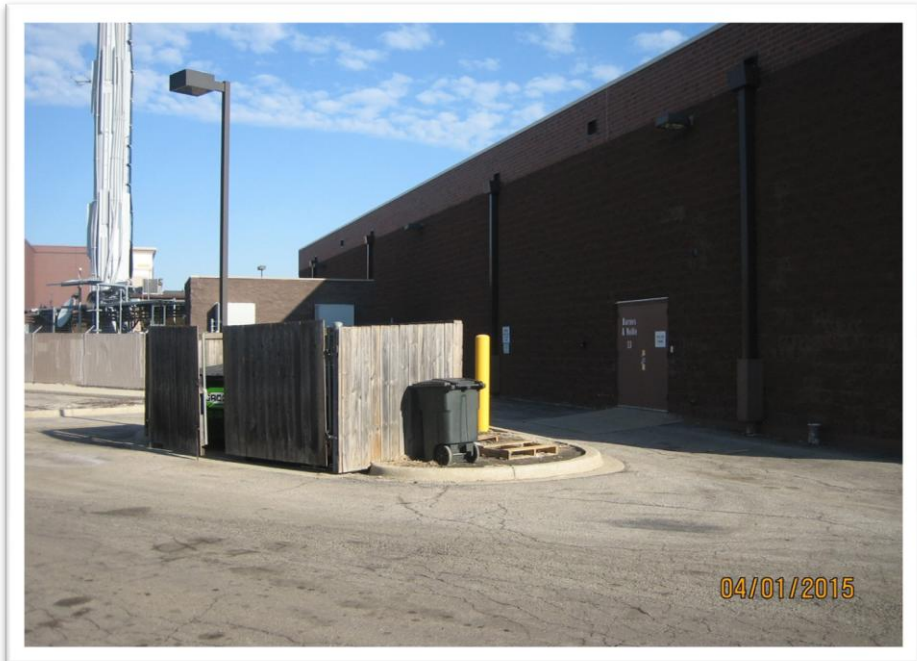
New Trash Enclosure at rear to match existing shown above.
