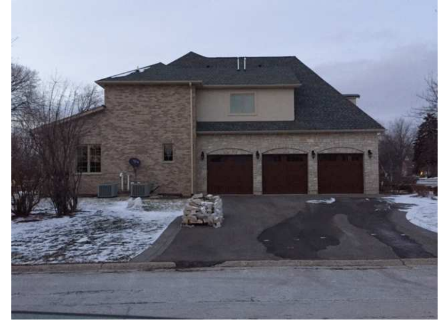
1606 N. Highland – South Elevation
