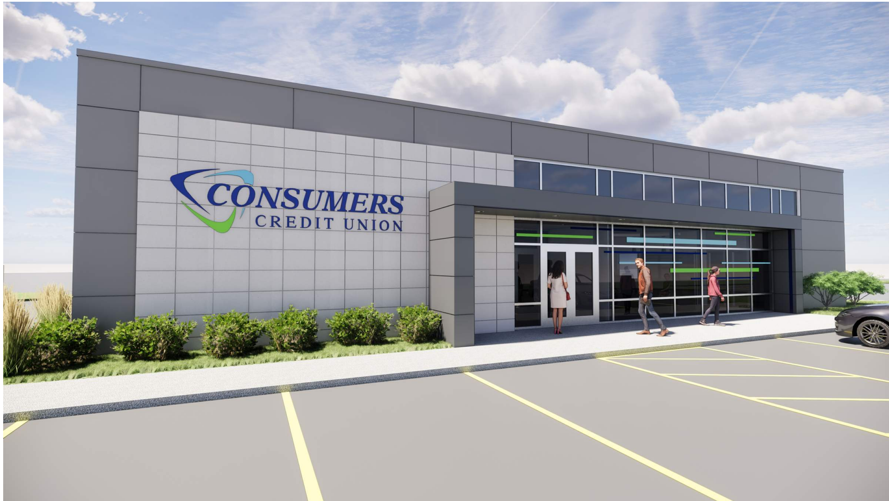
VIEW FROM SOUTHWEST
