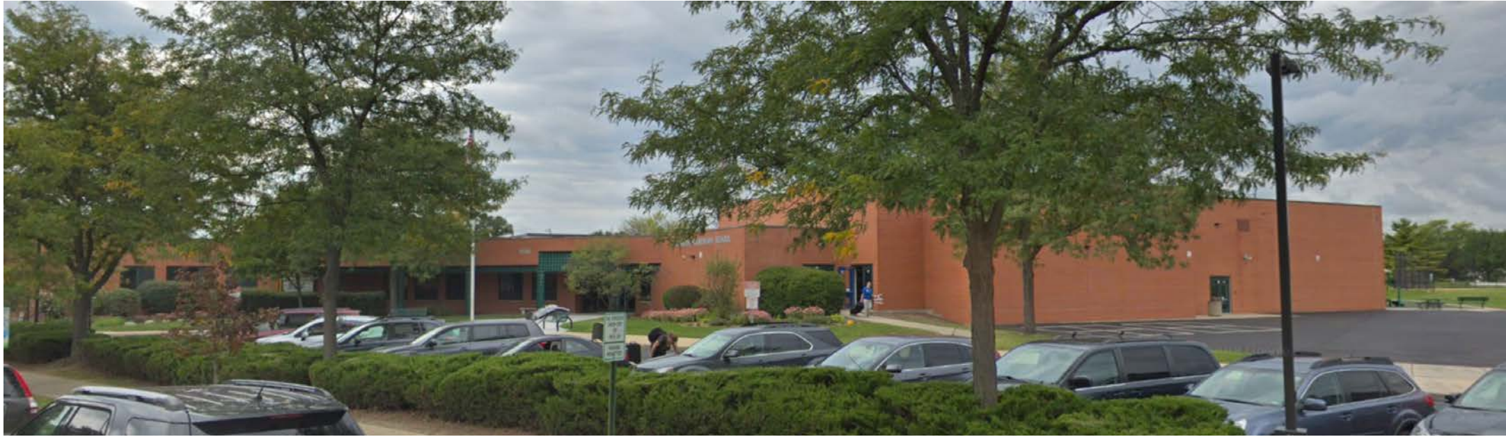
VIEW OF NORTH SIDE OF THE SCHOOL
