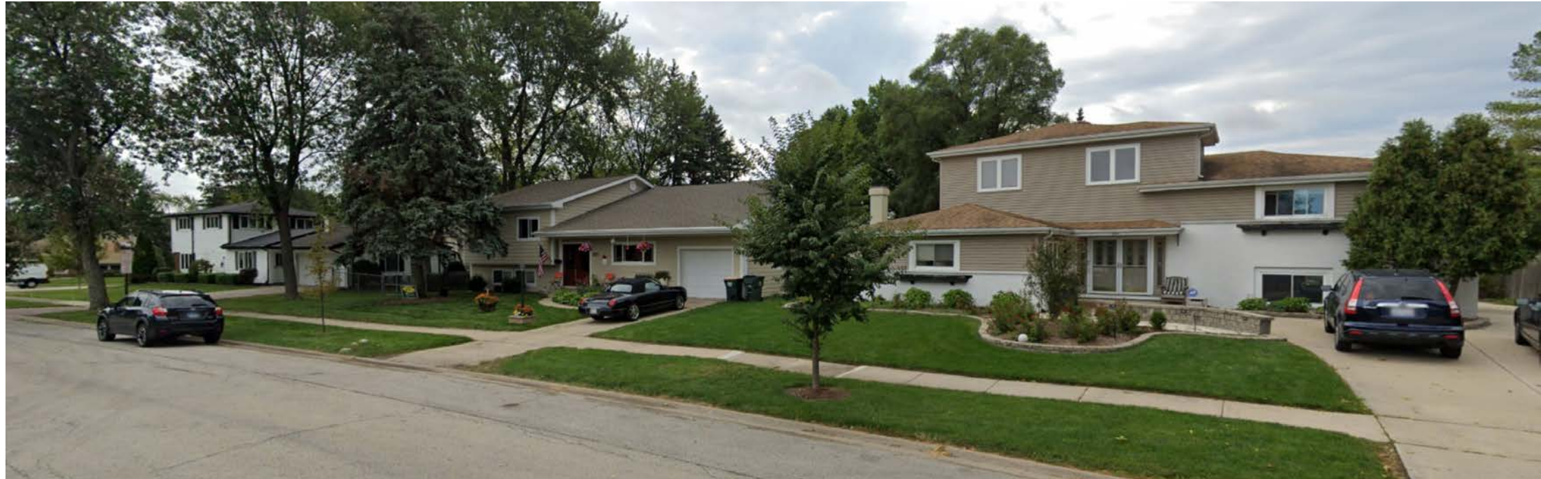
PROPERTIES AT THE SOUTHWEST SIDE OF THE SCHOOL - W. ROANOKE DR.
