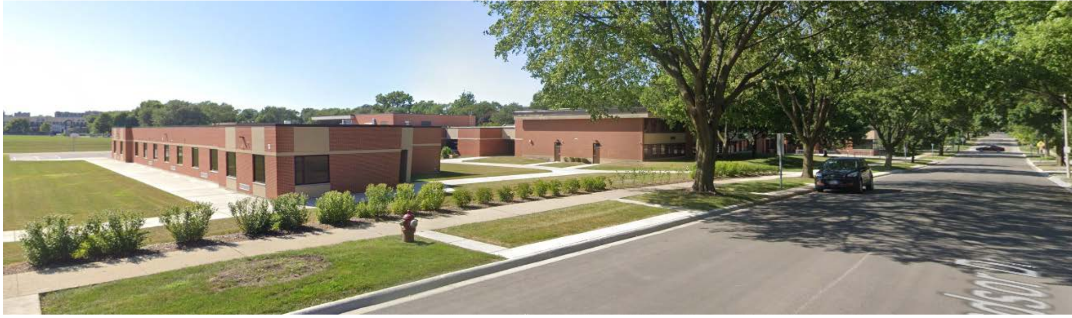
VIEW OF THE SOUTHEAST CORNER OF THE SCHOOL
