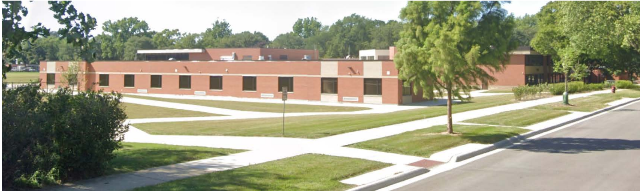
VIEW OF THE SOUTH SIDE OF THE SCHOOL
