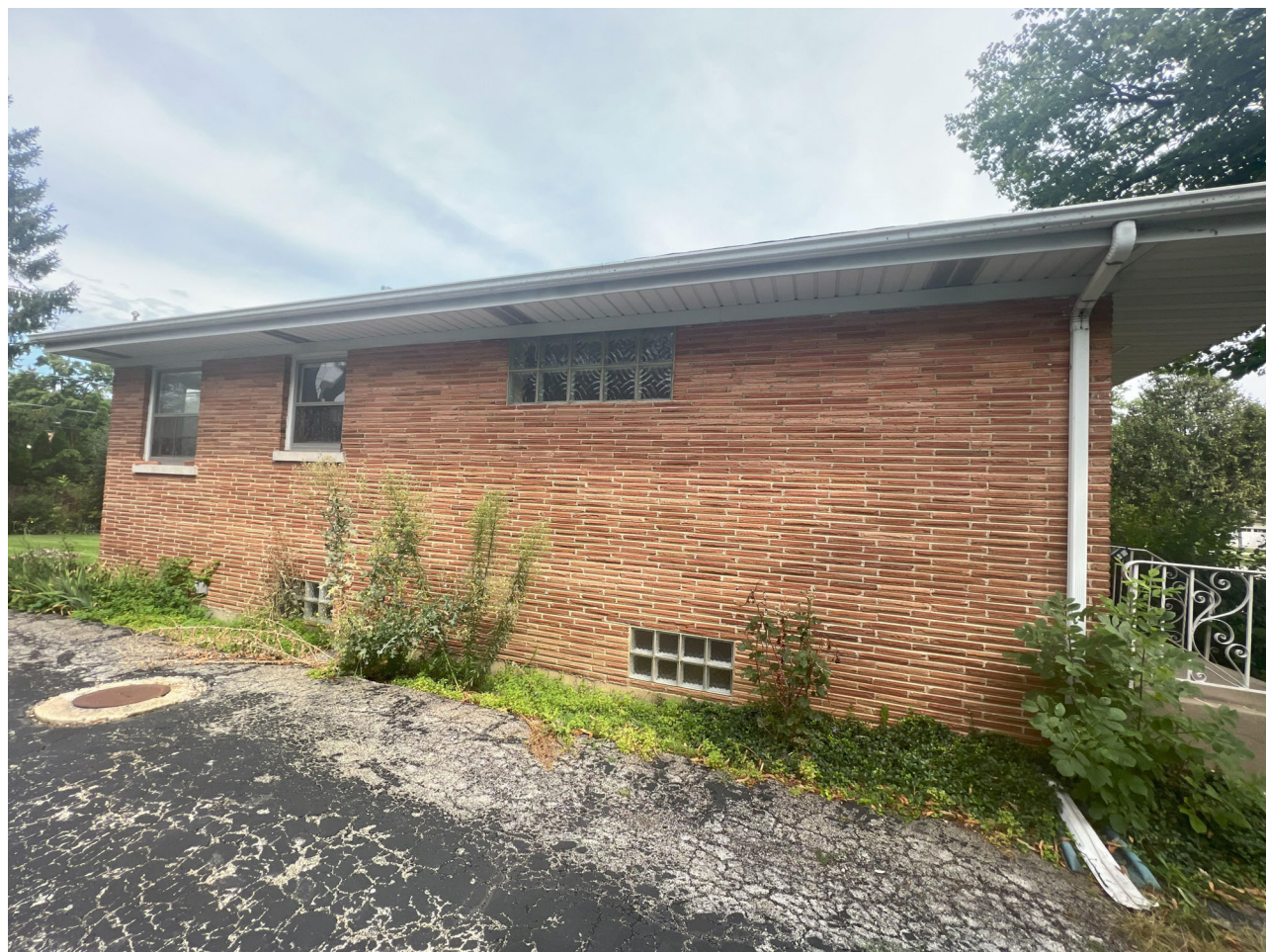
EXISTING HOUSE TO BE DEMOLISHED
