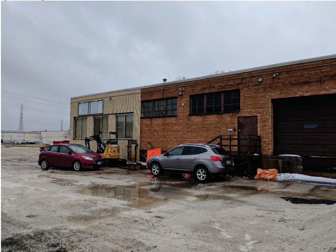
Existing Building at South End of Site
