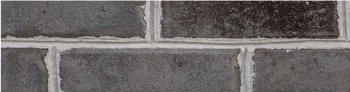
Brick Chimney – Palmetto Ashland
