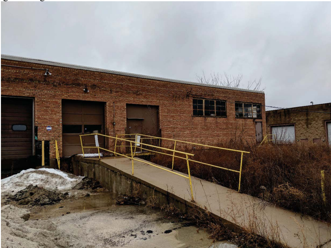
Existing Building at South End of Site
