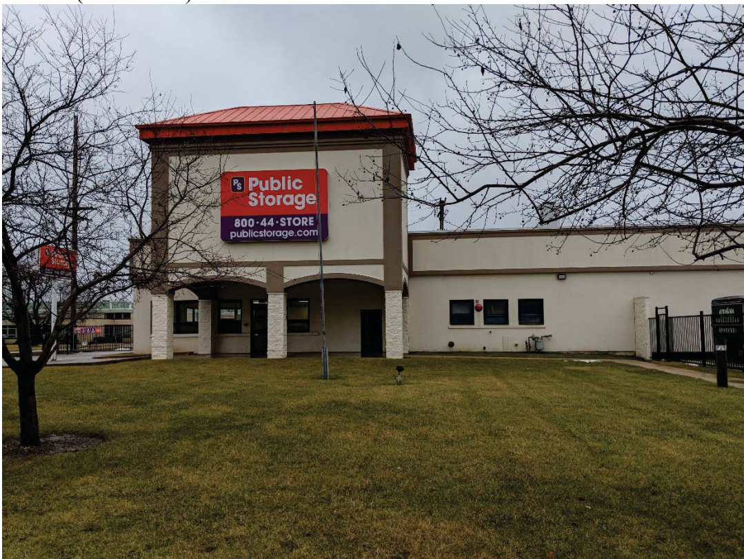
1600 E. Davis (East of Site)
