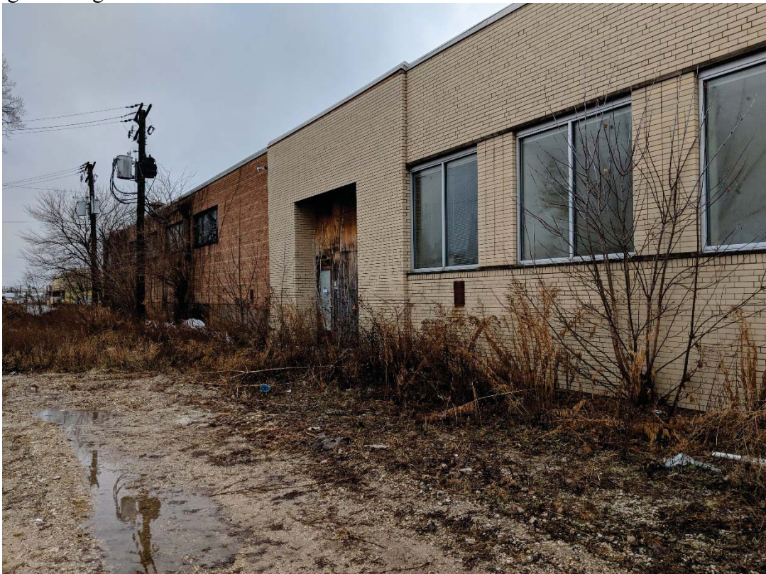
Existing Building at South End of Site
