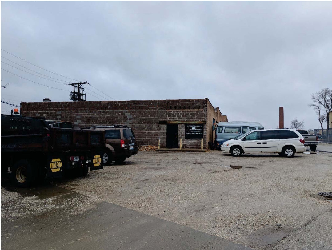
1442 E. Davis (East of Site)
