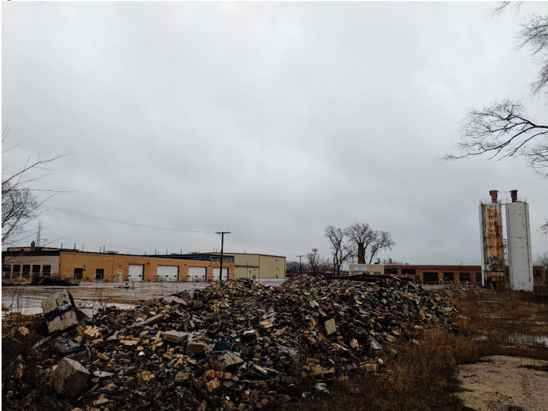
Existing Site – Southeast View
