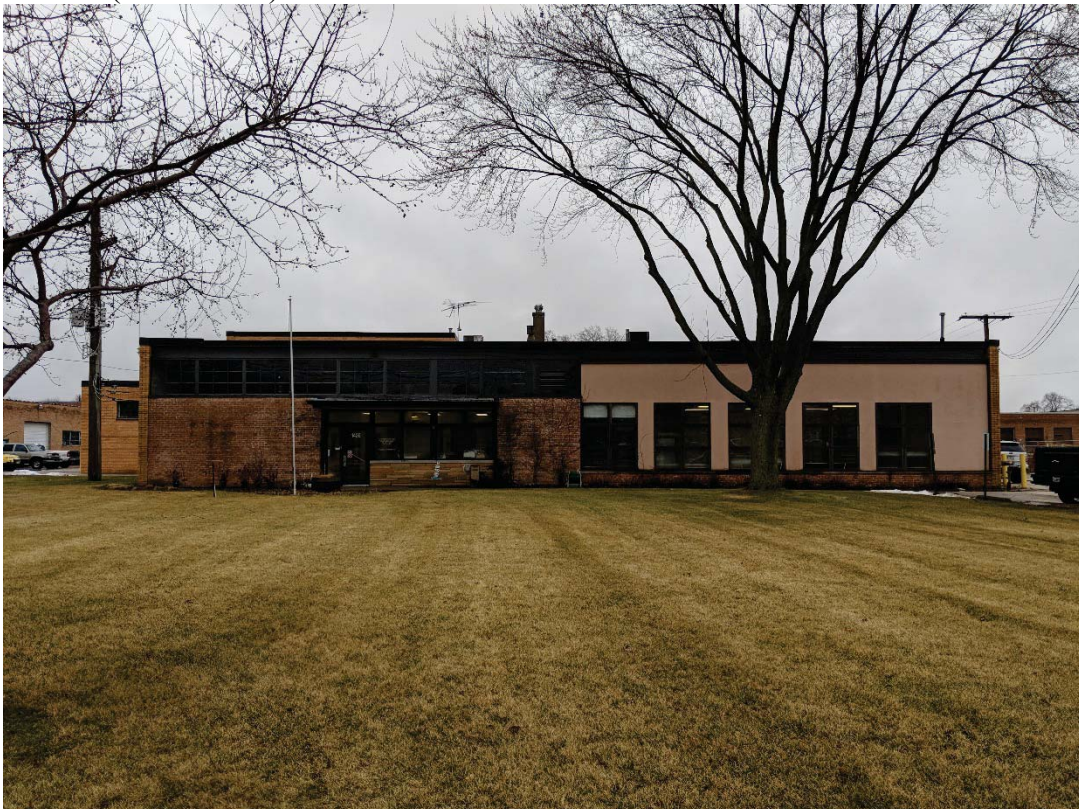
1436 E. Davis (East of Site)
