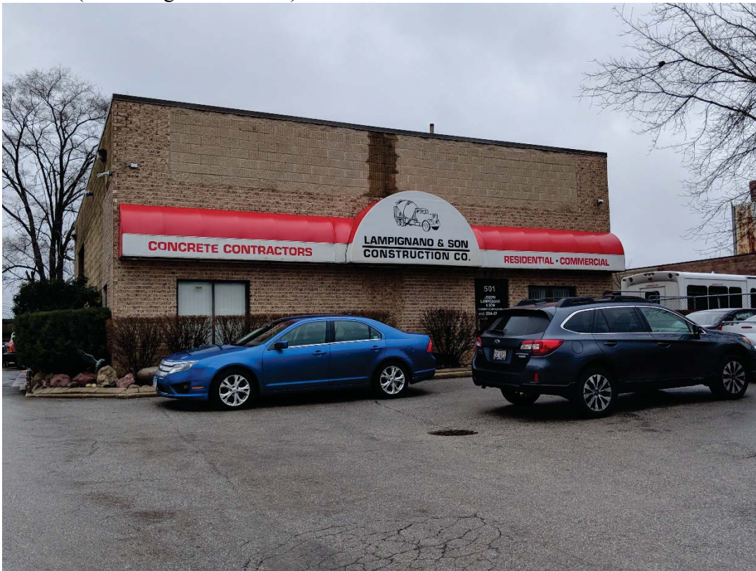
501 N. Arthur (Bordering Site to West)
