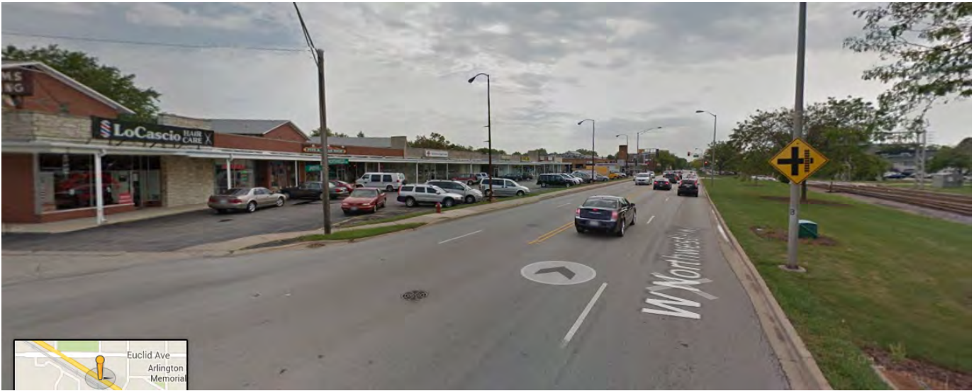
Looking back East at NWH / Ridge Ave
