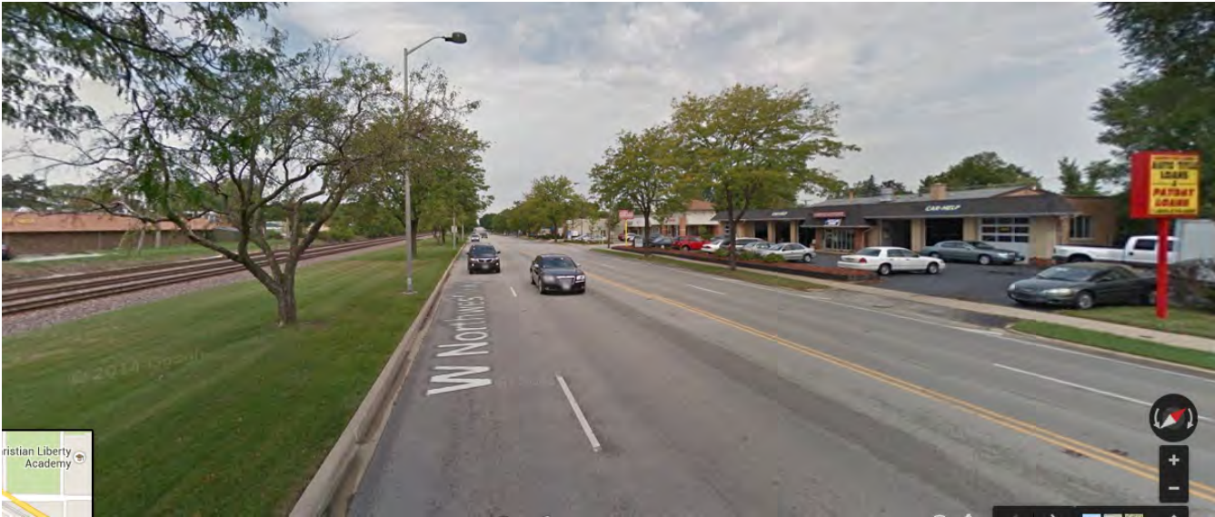
Looking West near Kennicott Ave
