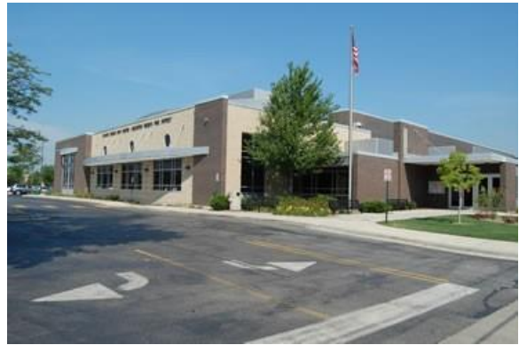
View of looking NW from Euclid / Ridge
