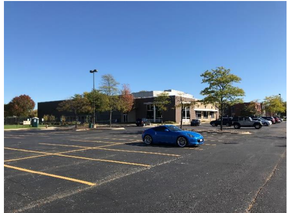
View looking east from south parking lot
