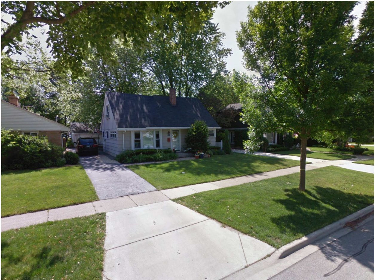
Photograph of Existing Structure
