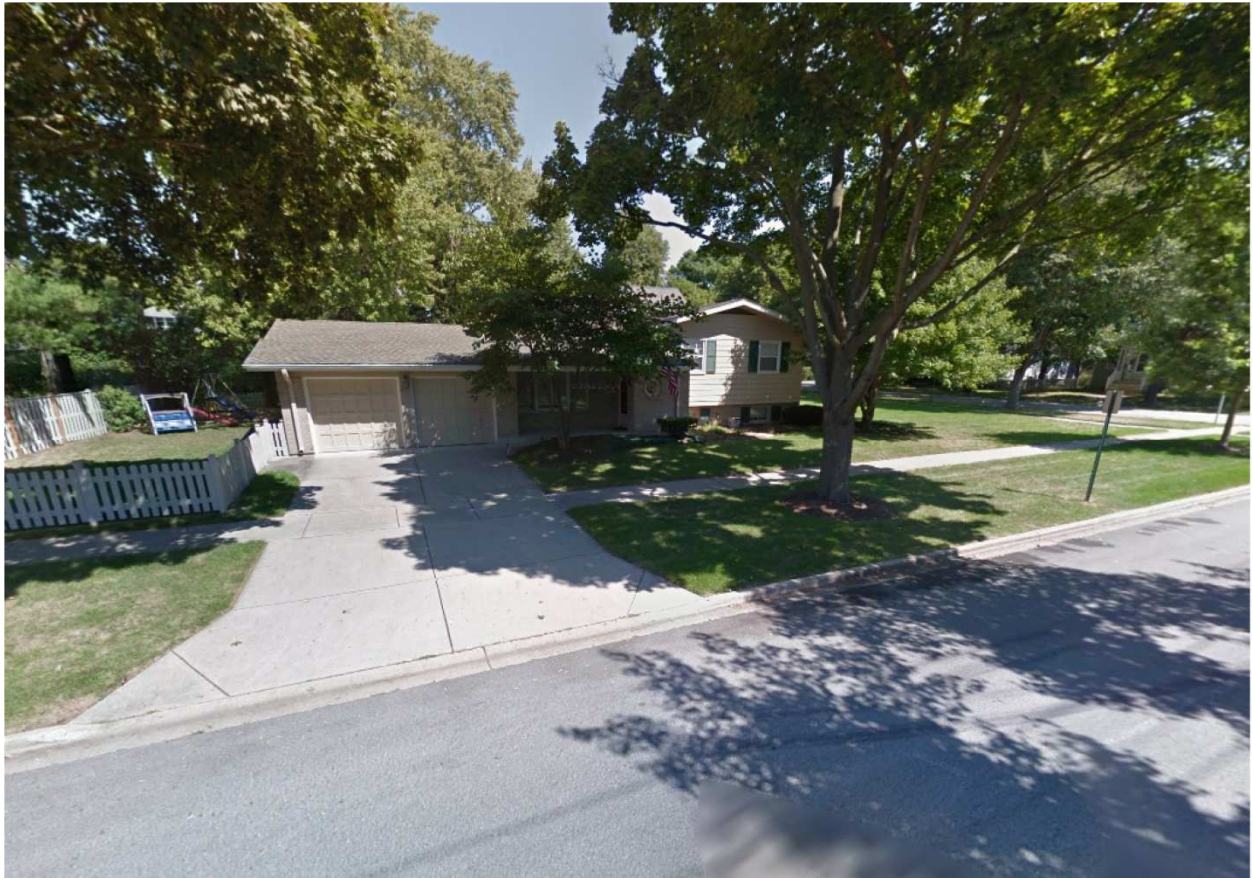
Photograph of Existing Structure
