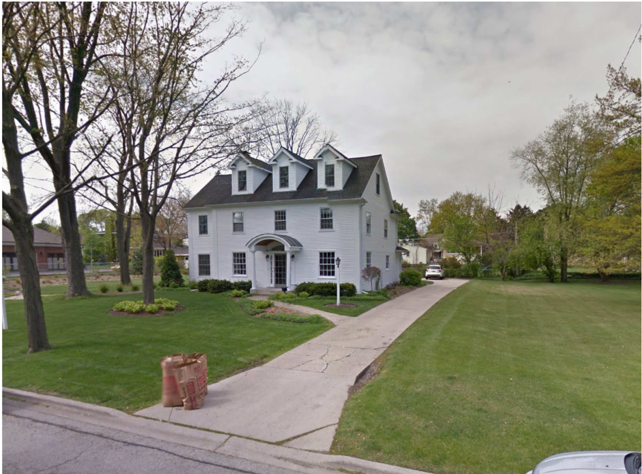
Photograph of Existing Structure
