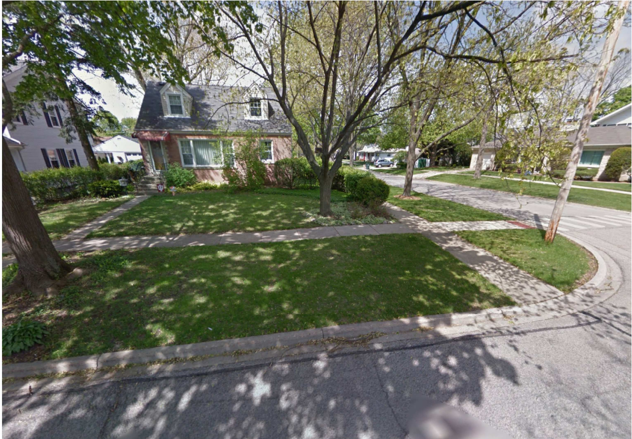
Photograph of Existing Structure
