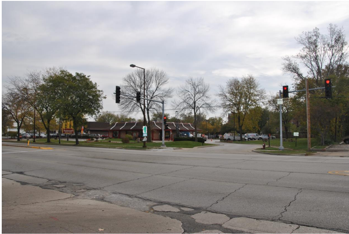
Intersection of Dundee Rd and McDonald's/Oberweis Dairy access drives
