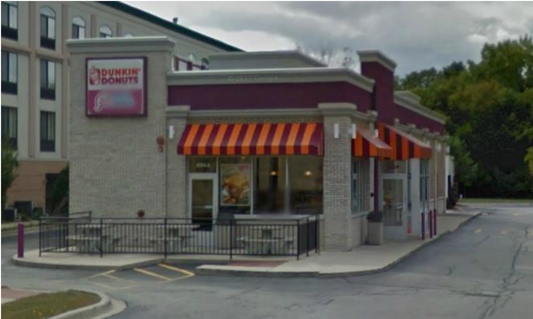
Photo 2. Existing Dunkin Donuts restaurant located at 2106 S. Arlington Heights Road in Arlington Heights.
