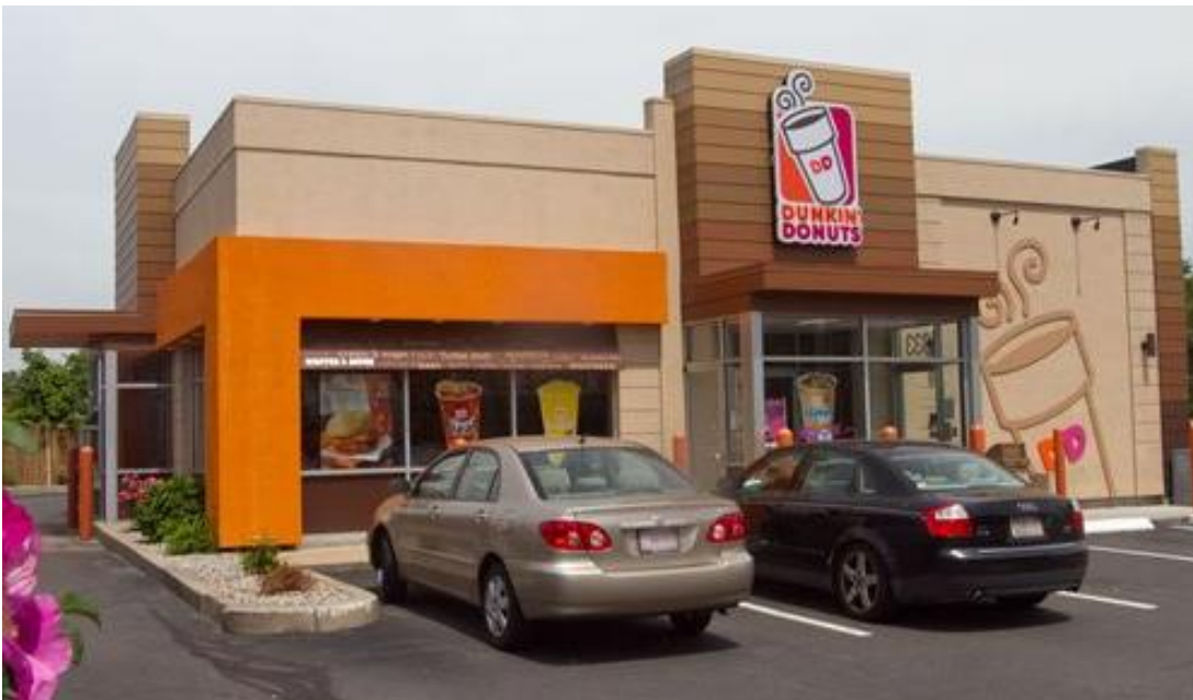
Photo 3. Similar new Dunkin Donuts prototype restaurant with EIFS walls and mitered siding corners.
