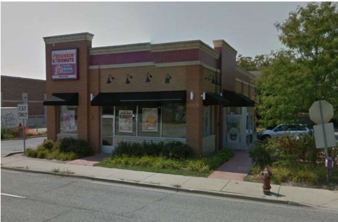
Photo 1. Existing Dunkin Donuts restaurant located at 122 S. Arlington Heights Road in Arlington Heights.
