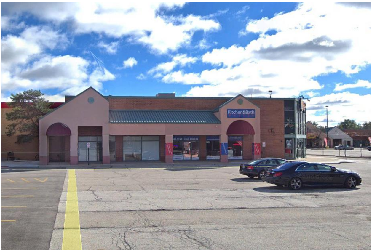
Adjacent building to the North of Bif Furniture (western aspect)
