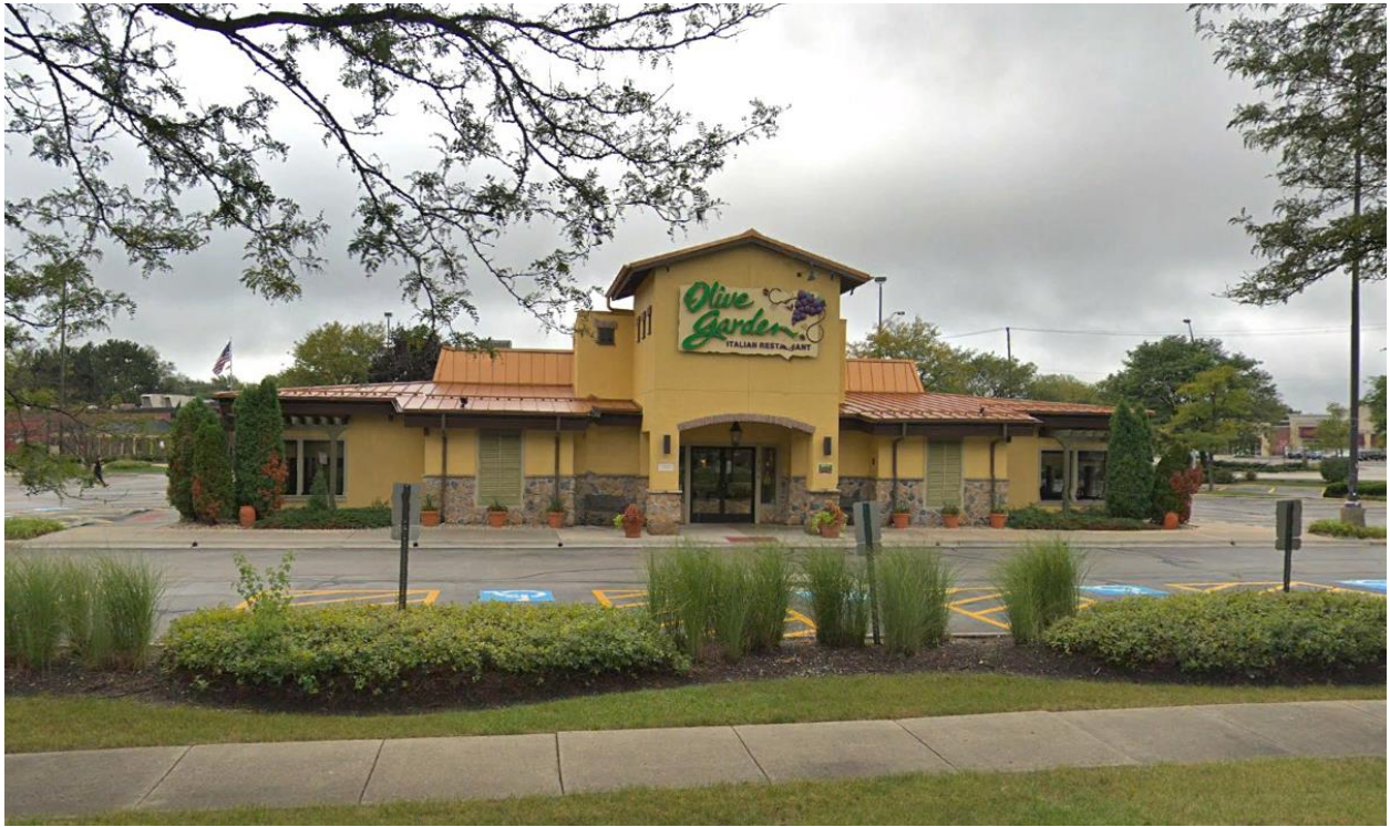
Existing Olive Garden restaurant outlot building
