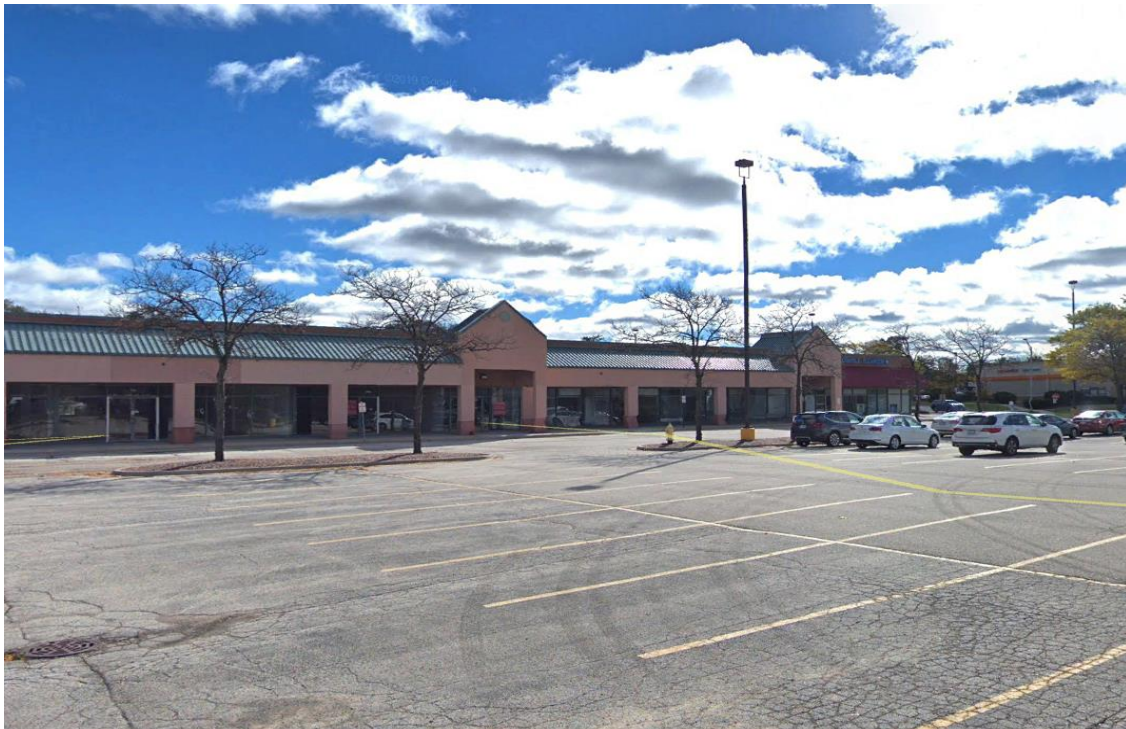
Existing Building to the South of Bif Furniture (to remain)
