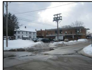
SUBJECT PROPERTY REAR ELEVATION 413 S. ARLINGTON HEIGHTS RD.
