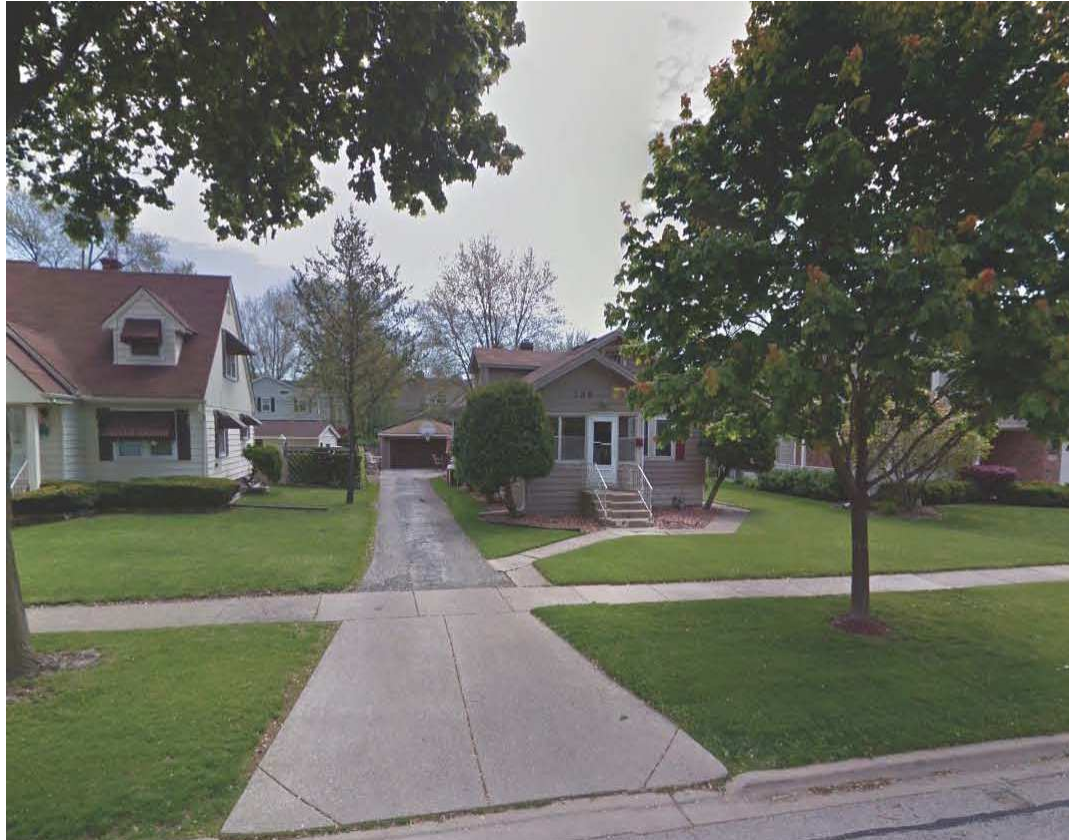
Photograph of Existing Structure
