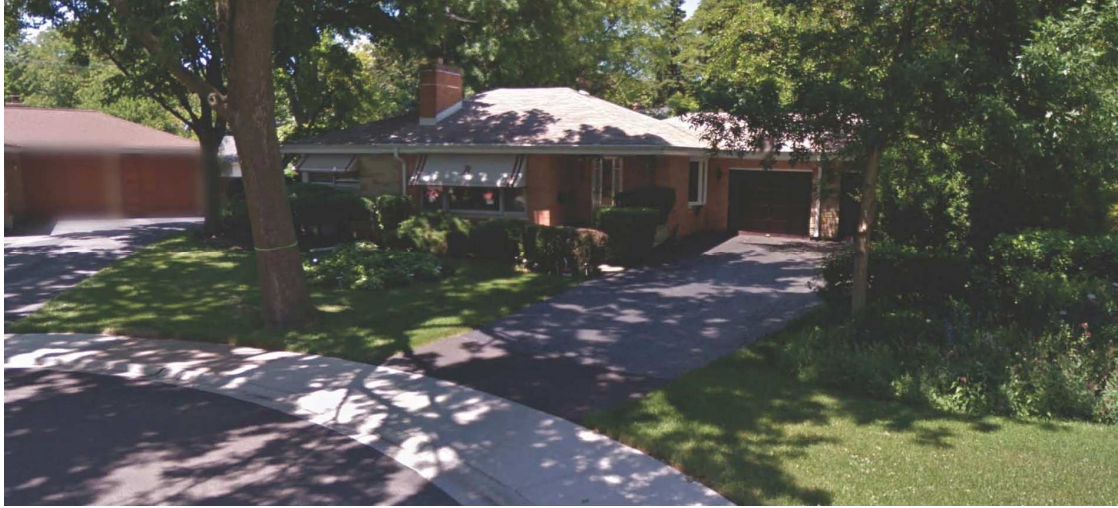
Photograph of Existing Structure
