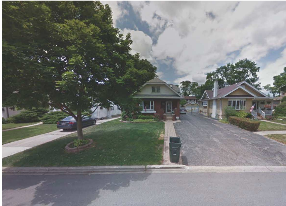
Photograph of Existing Structure
