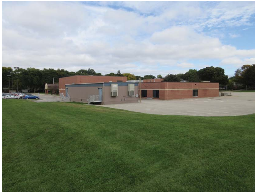
VIEW - AT SOUTHWEST CORNER OF SCHOOL
