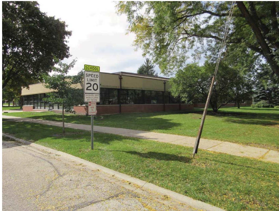
VIEW - AT NORTHEAST CORNER OF SCHOOL
